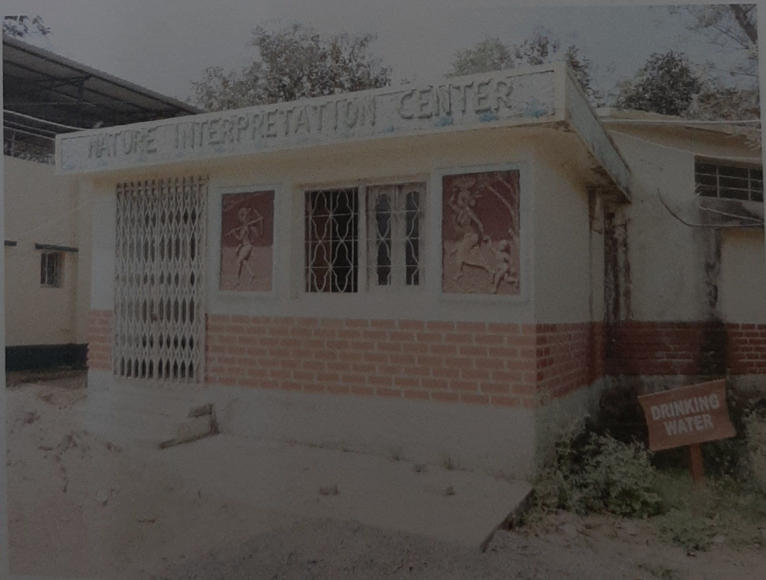
Nature Interpretation Center under construction
