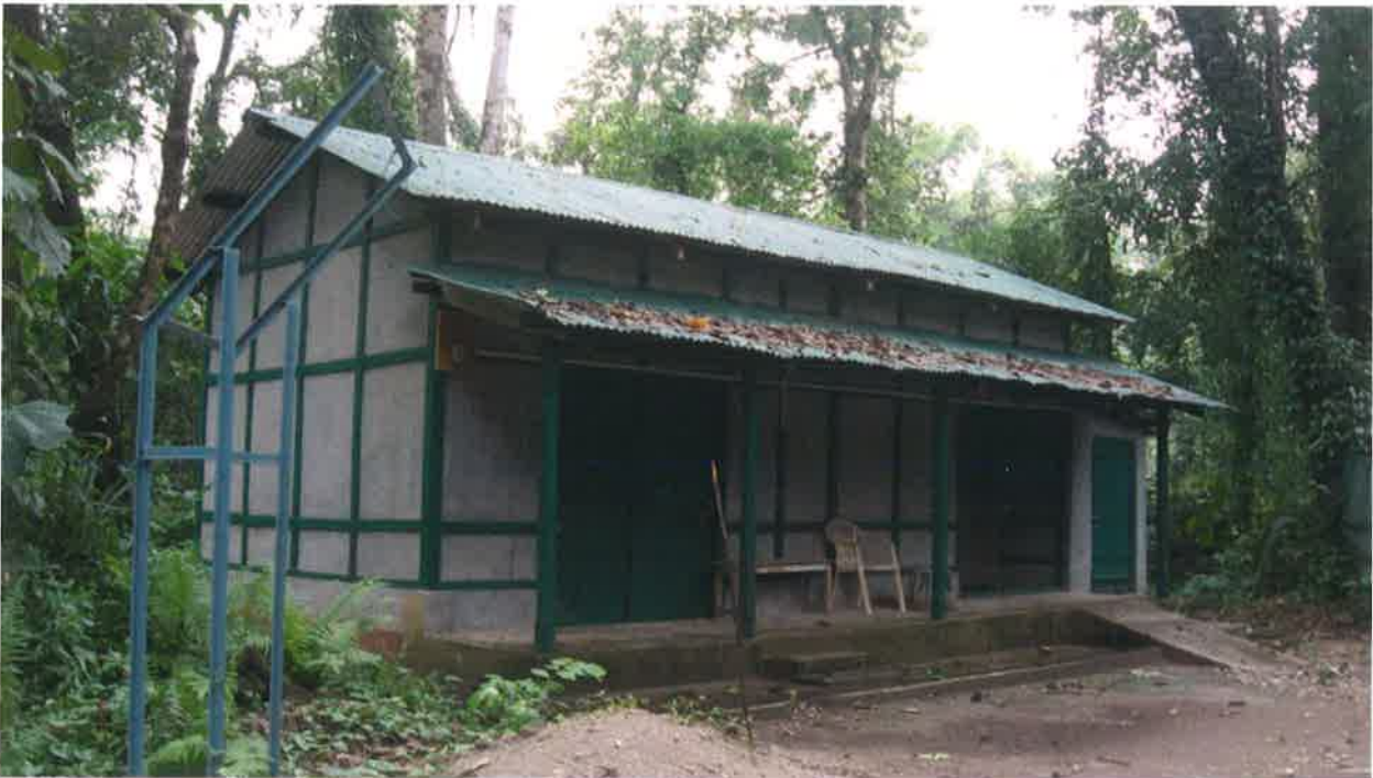
Fig: Support building with stores, kitchen, keeper room and examination room.
