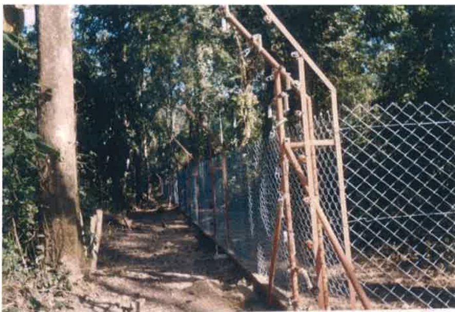
Fig: The solar fencing around the shelter area.
