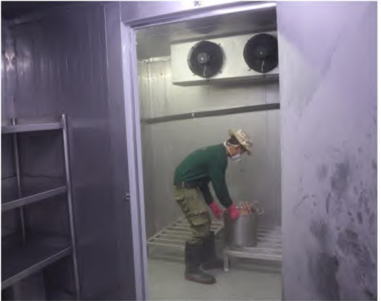
Figure 2.12: Cold Food storage area of GZRRC
