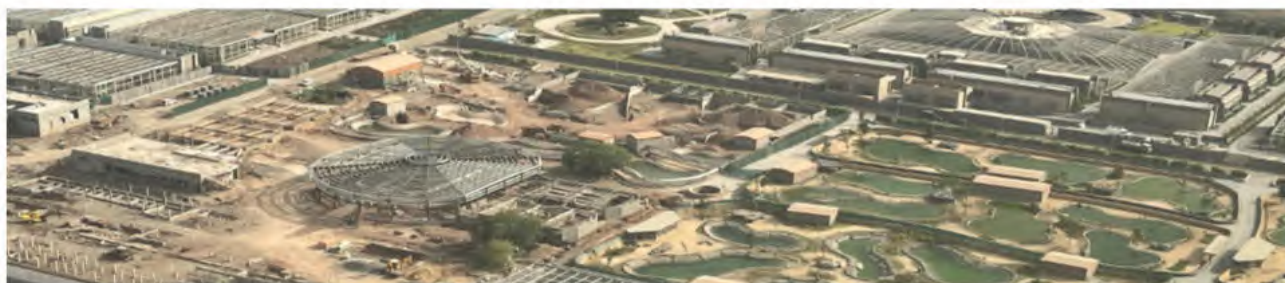
Figure 2.1: Aerial Veiv of GZRRC Facilities Under Construction
