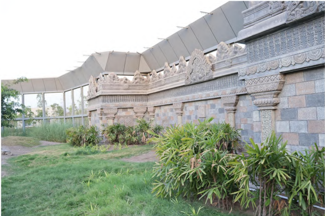
Figure 2.5: Top-Open Enclosure for Large Felids with Overhang and Power-fence at the Rescue and Rehabilitation Facility of GZRRC
