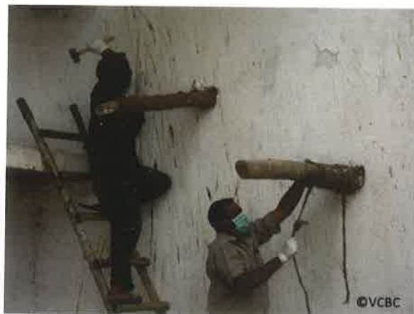
Repair of perches
