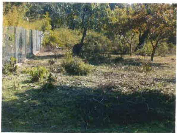
Chain link perimeter fence bordering the centre
