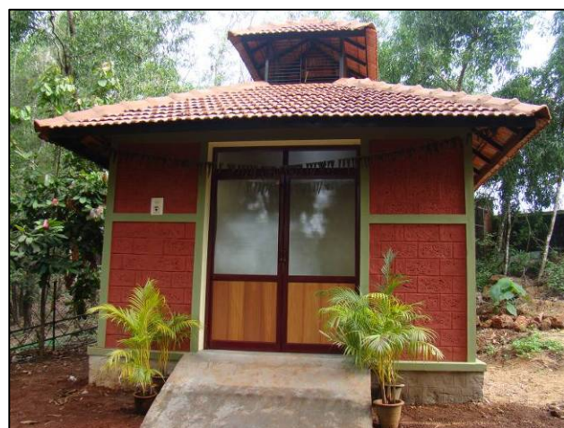
Newly Constructed Post-mortem Building
