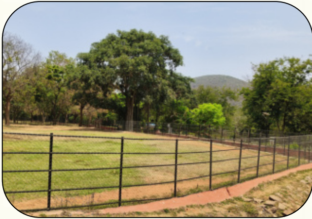
1/2"x1/2" -12 Gauge Chain link Mesh to Giraffe Night House in IGZP, Vsp During 2024-25
