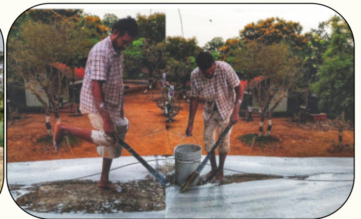
Cool roof painting of an animal night enclosure
