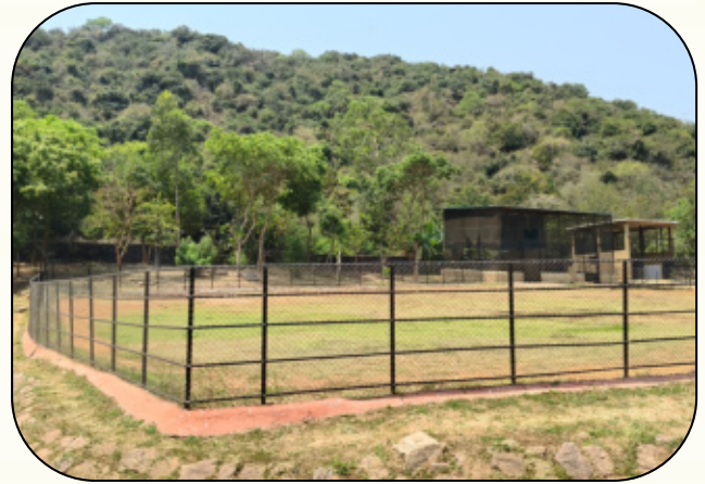
1/2"x1/2" -12 Gauge Chain link Mesh to Giraffe Night House in IGZP, Vsp During 2024-25
