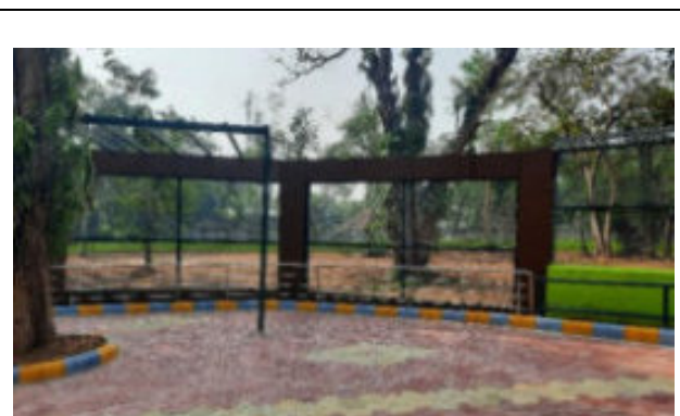
New Zebra enclosure on near completion
