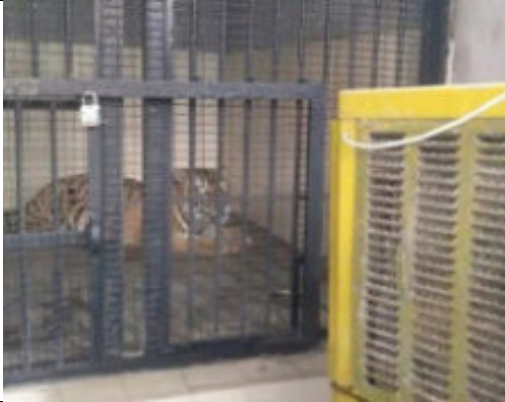
Desert coolers installed at the keeper gallery for large cats as summer management action
