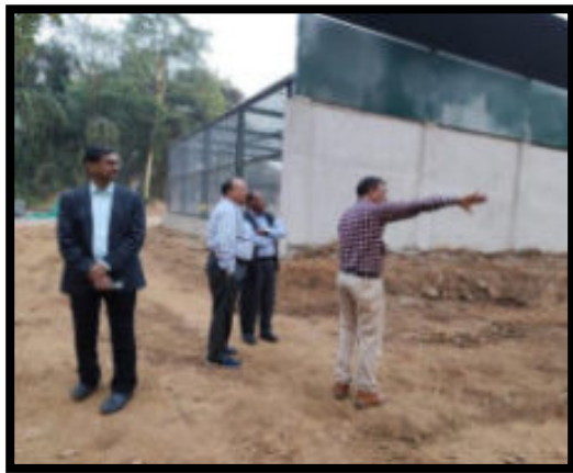
Visit of ZVHAC team at the construction site of Lion & Tiger
