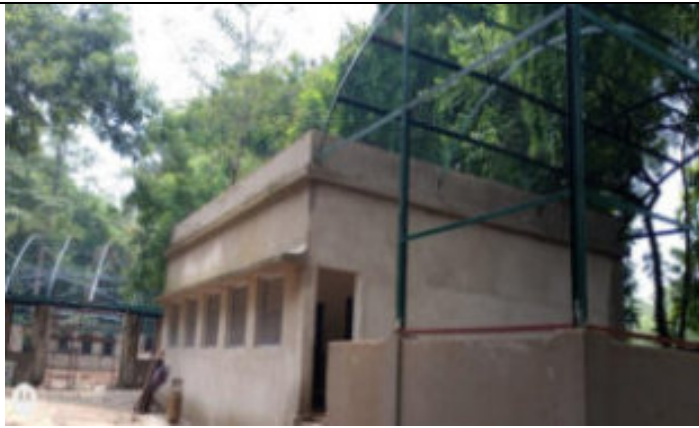
Under construction Butterfly Arena at the new site
