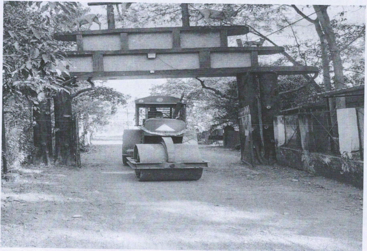
Repairing of Morrur Road from Main Entrance Gate to Zoo Office
