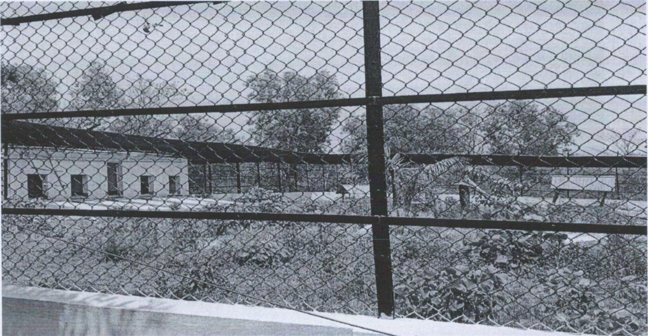
Renovation of Leopard Enclosure
