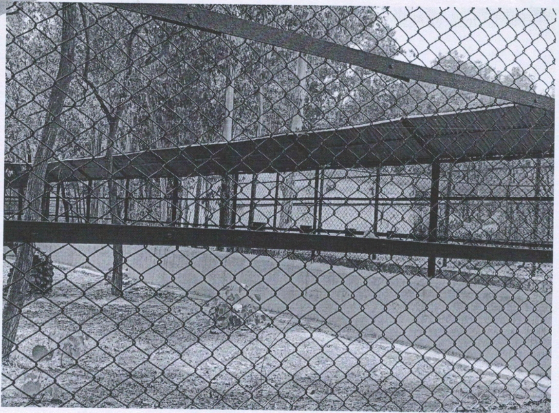
Renovation of Hyena Enclosure
