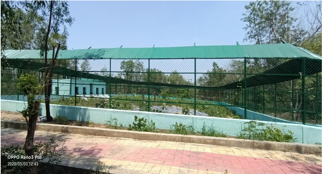
Construction of Leopard Enclosure
