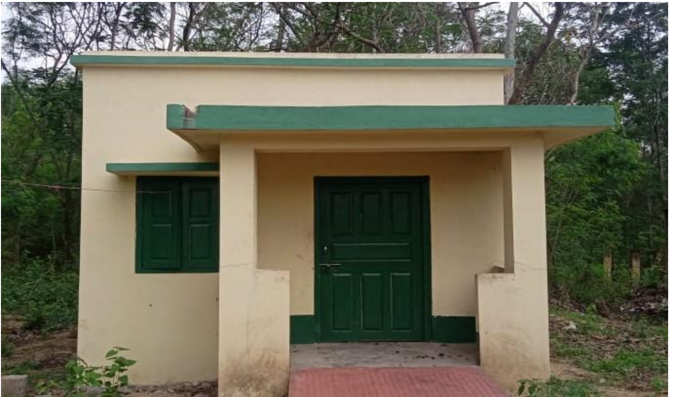
Construction of Post Mortem room
