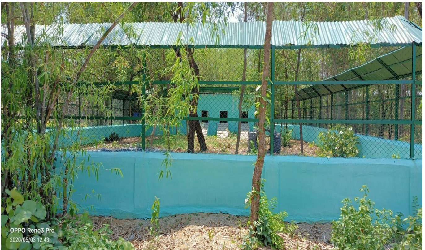
Construction of Hyena Enclosure
