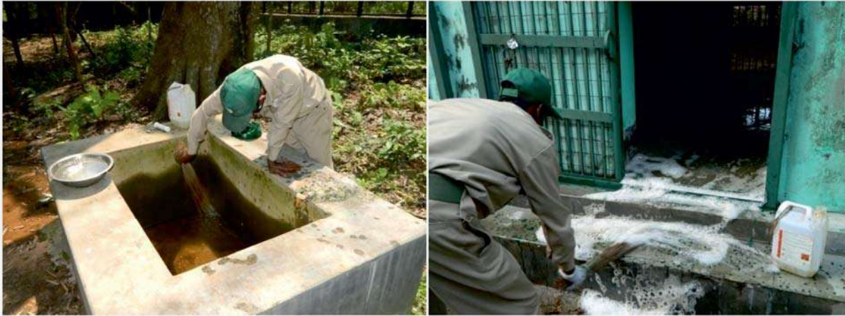
Routine cleaning of water tanks with disinfectant
