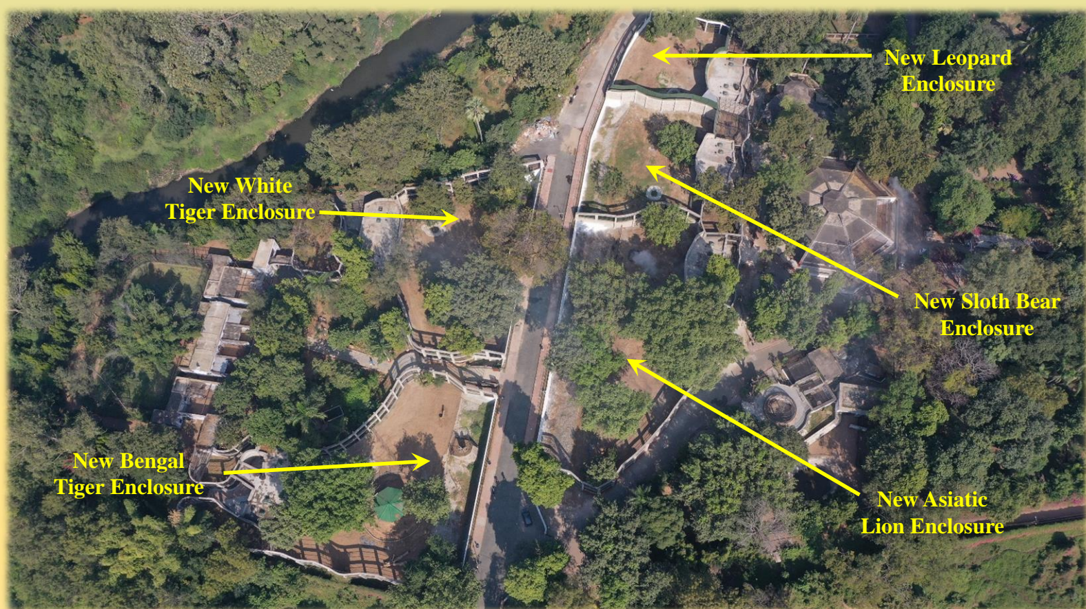
Drone View – All New Moat Enclosures E-Inaugurated on 1 st December 2020
