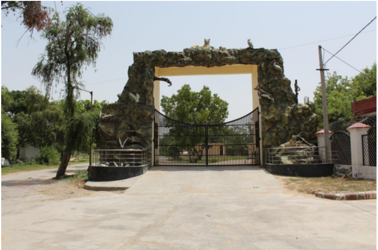
Main Gate of the Rohtak Zoo
