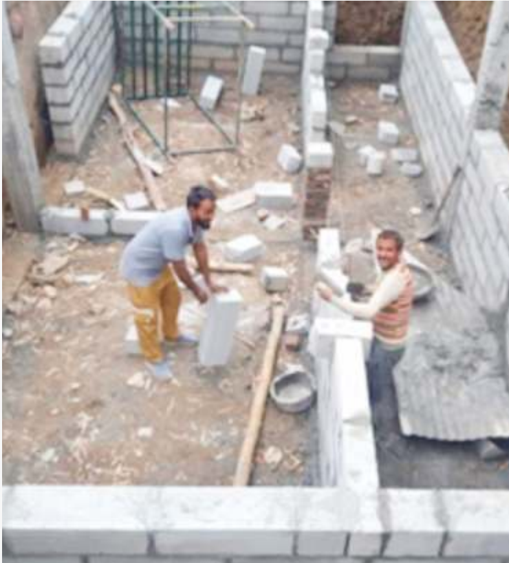
New bear night shed under construction
