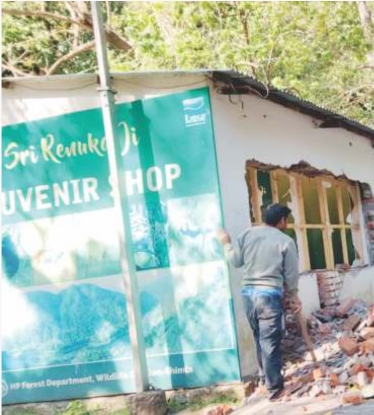
Souvenir shop under renovation
