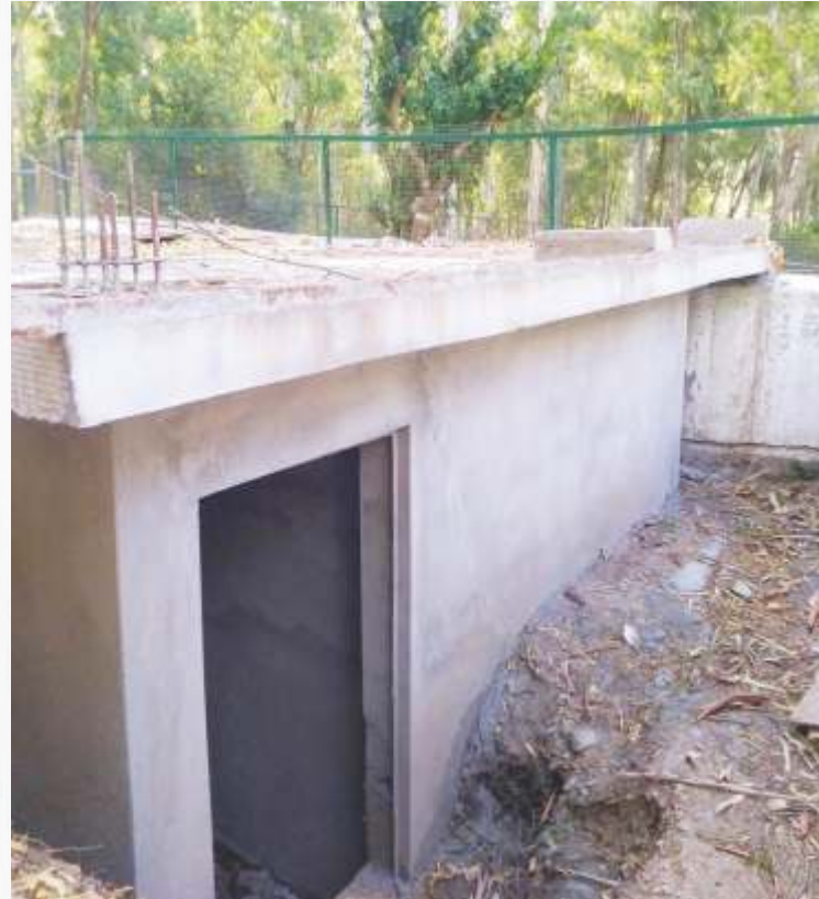
Constructed new bear night shed
