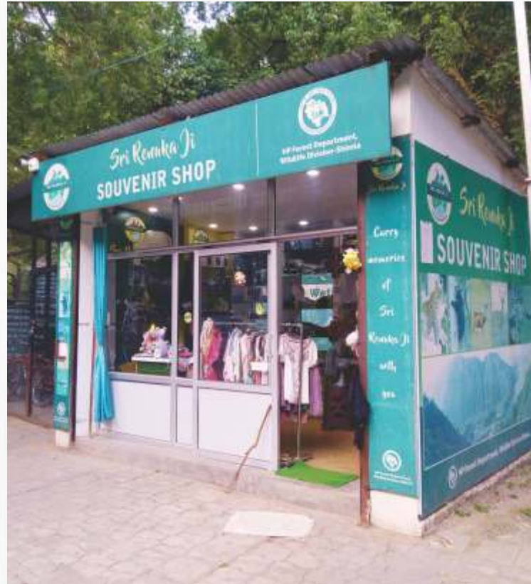
Renovated Souvenir shop
