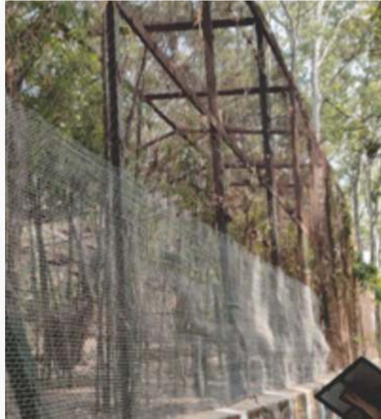
Aviary enclosures secured with fine-mesh fence
