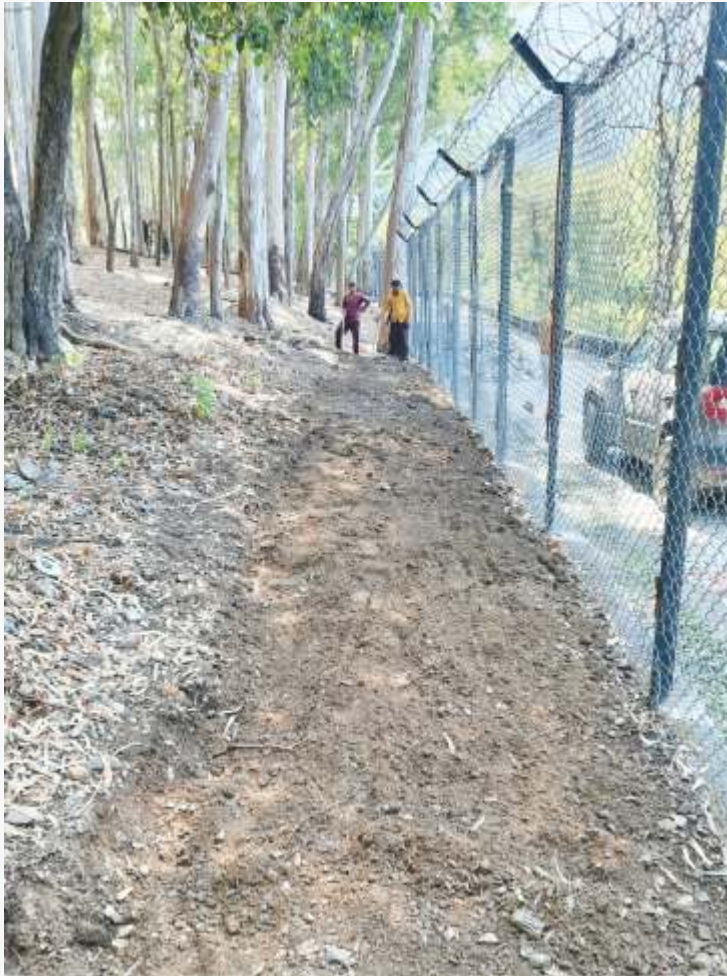
Alternate path under construction
