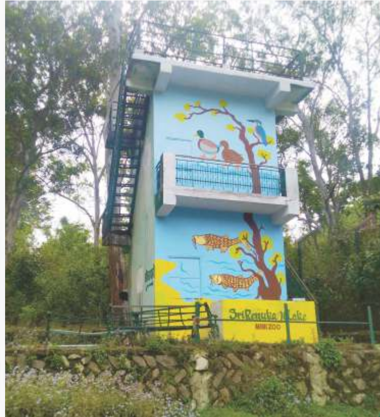
Watch tower after renovation
