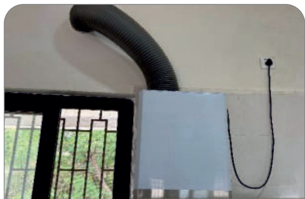
Chimney in Non-Veg Section
