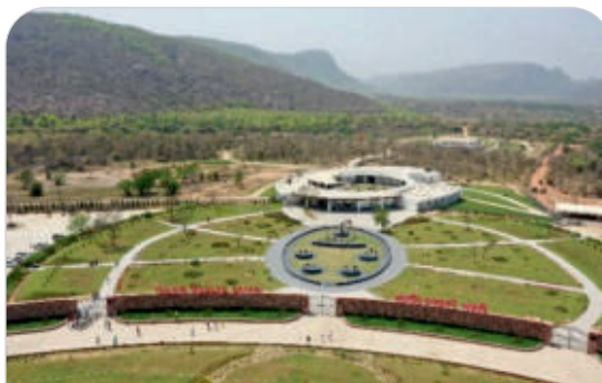
Aerial view of Reception and Orientation Zone
