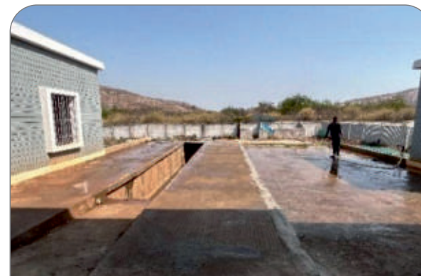
Bus Washing Area
