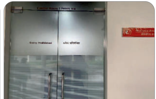
Entrance of Control Room
