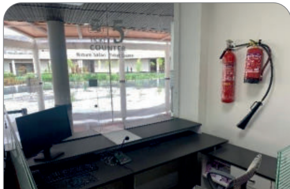
Ticket counter Fire Safety
