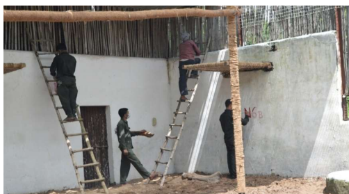
Scrubbing and disinfecting walls with lime
