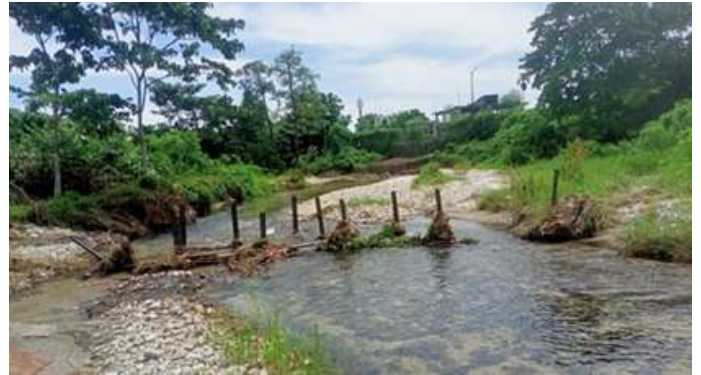
MS joists constructed across river
