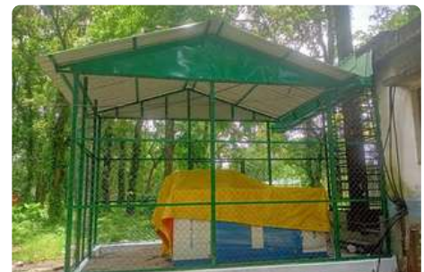
Extension of Generator Room at NBWAP
