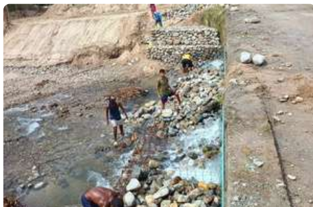
De-siltation of Jhora (Part-I) at NBWAP
