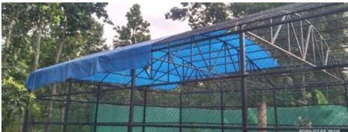
Tarpaulin cover at lion shelter
