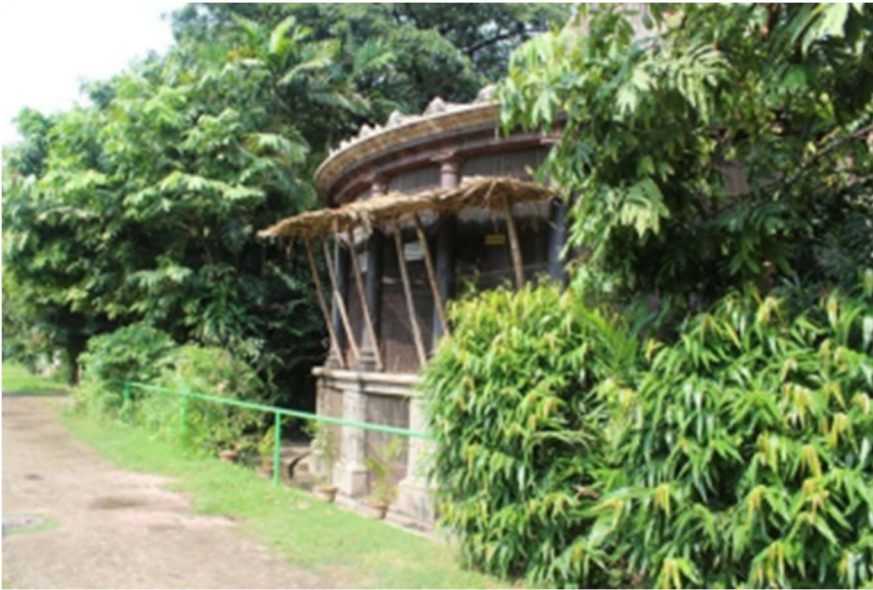
The heritage cage structures.
