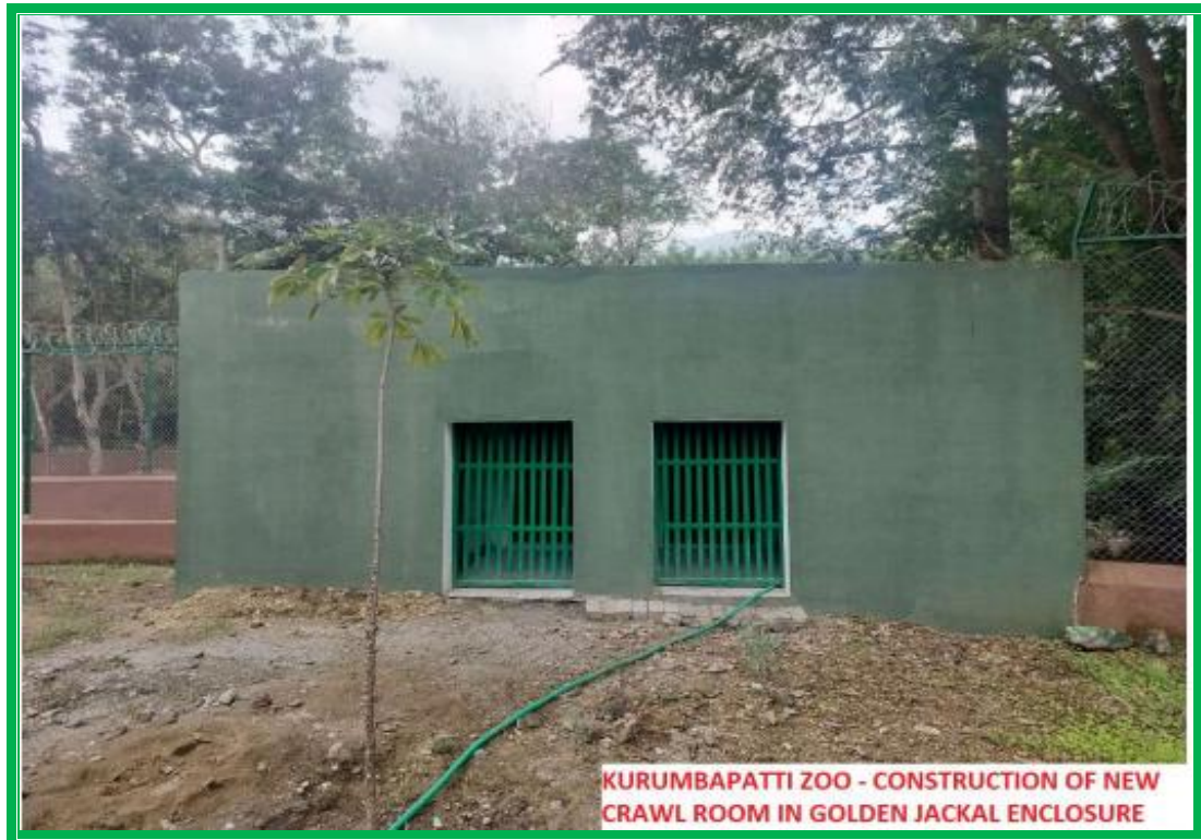
Construction of Kraal building for fox enclosure at KZP
