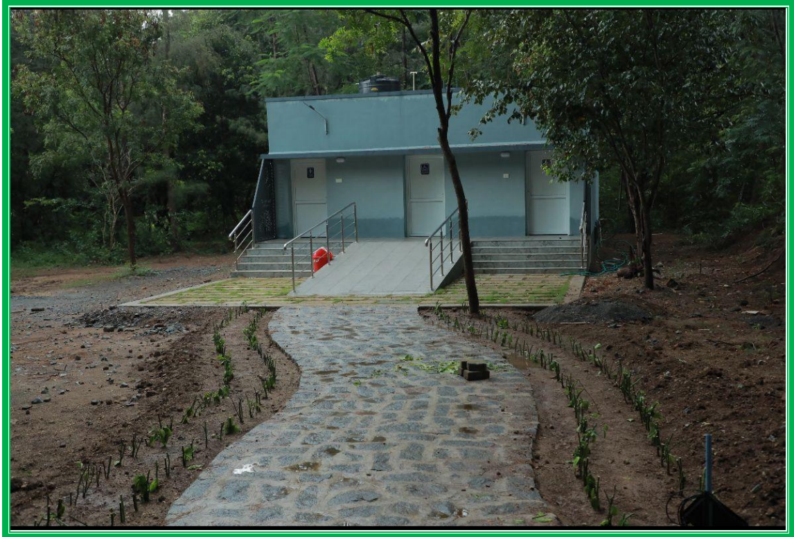
Construction of New Combined gents and women's toilet at KZP
