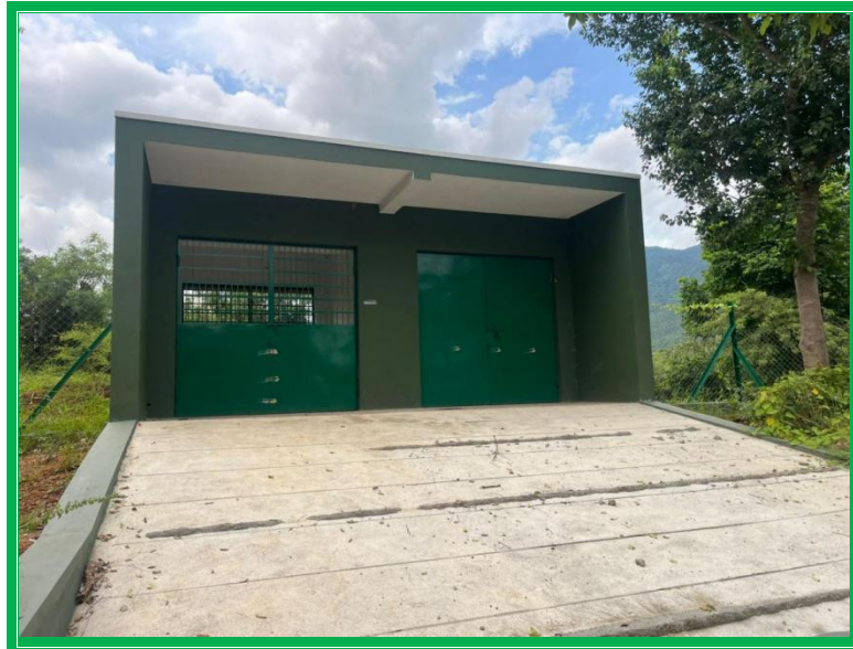
Construction of kraal Room for Nilgai enclosure at KZP
