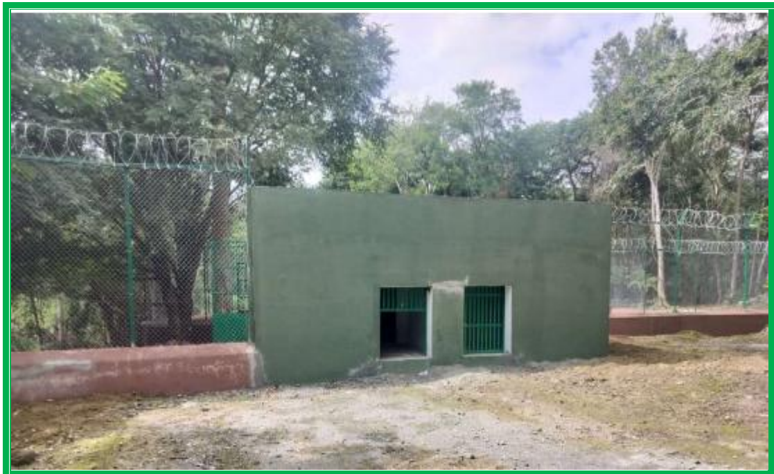
Construction of Kraal Building for jackal enclosure at KZP
