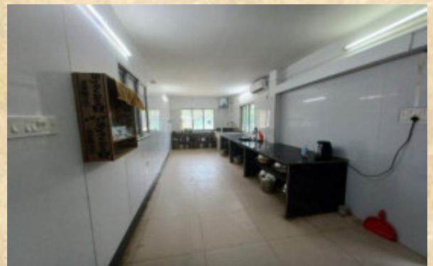
Renovation work of Food Store
