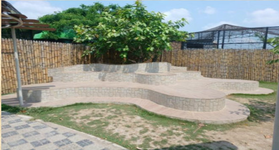
Construction of Sitting Platform near Gibbon enclosure
