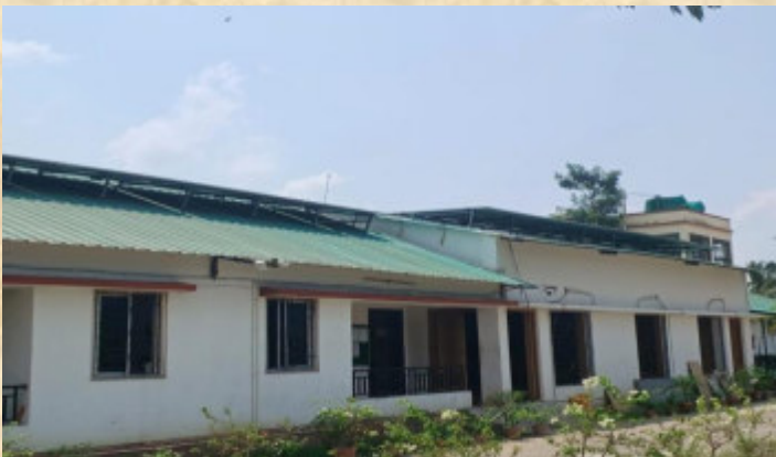
Supply and Installation of 50 KWP roof top Solar power plant ( Grid Mode)
