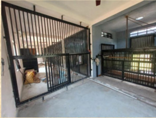
Construction of Night Shelter of Tiger Enclosure
