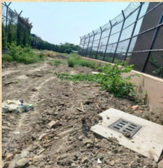
Construction of sewerage & drainage system, phase-II
