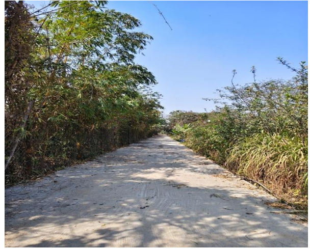
Extension of service path by concrete pavement from hippo enclosure to emergency gate beside lion enclosure (L-650m W-3.8m)
