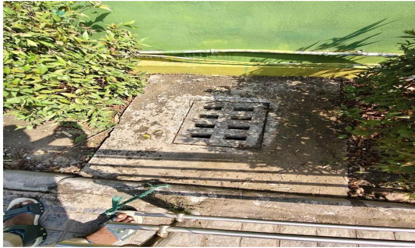
Land development and drainage work for Red-tail Monkey Enclosure
