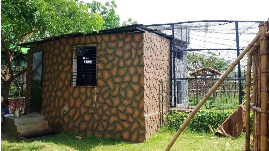
Additional works for Hoolock Gibbon Enclosure and Night Shelter
