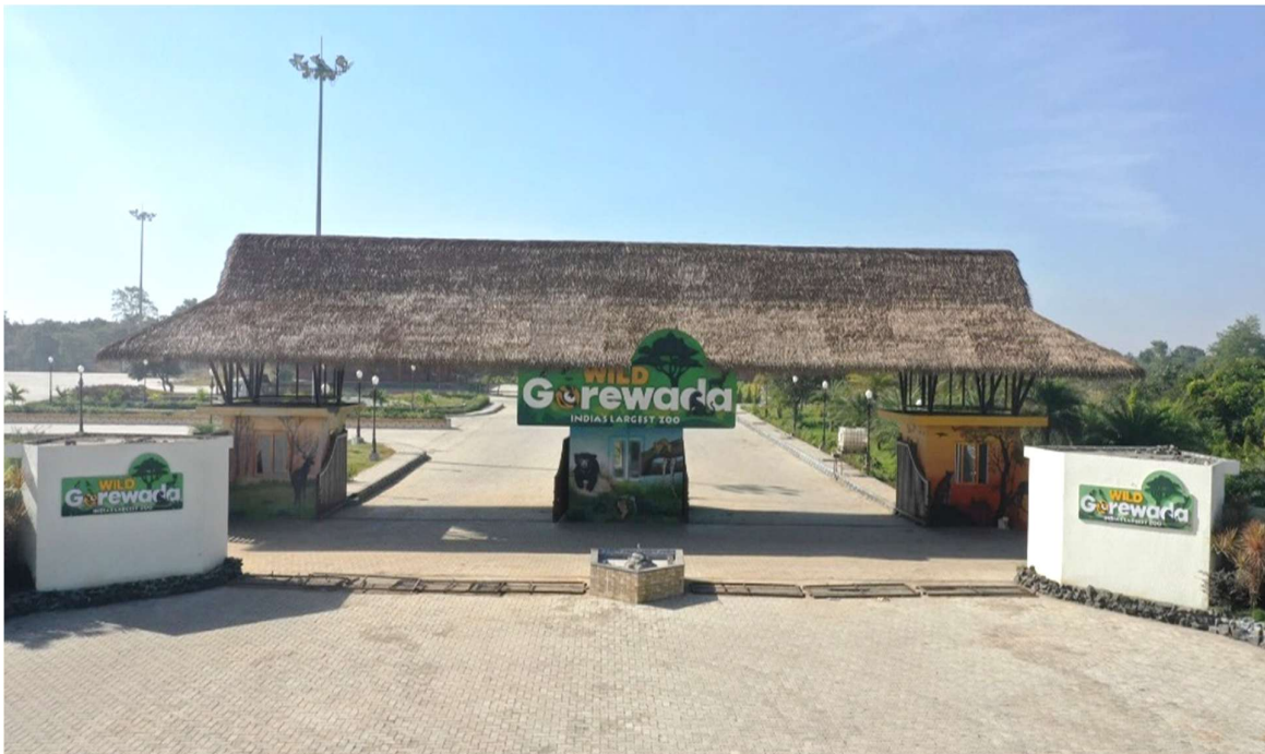
Figure 2: The Entry Gate
