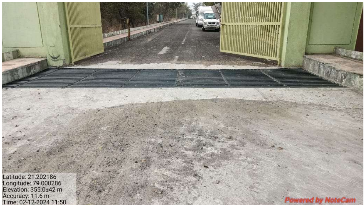
Cattle proof barrier at the Rescue Centre
