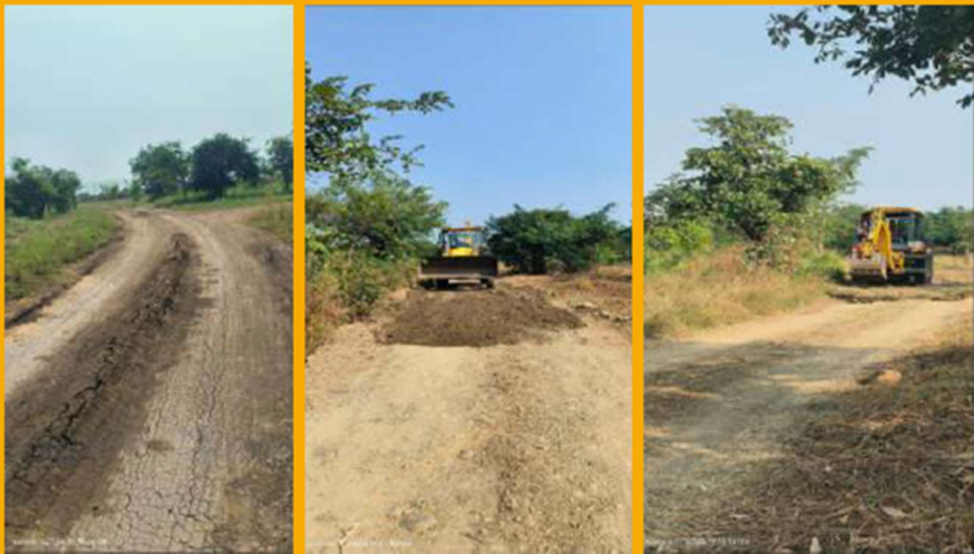
Road Repair and Maintenance in Gorewada Reserve Forest before opening it to visitors after Monsoon.
