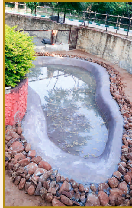
Renovation of Crocodile pond
