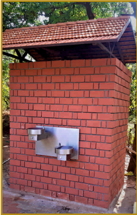
RO Drinking water unit
