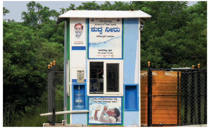
RO Drinking Water Plant
