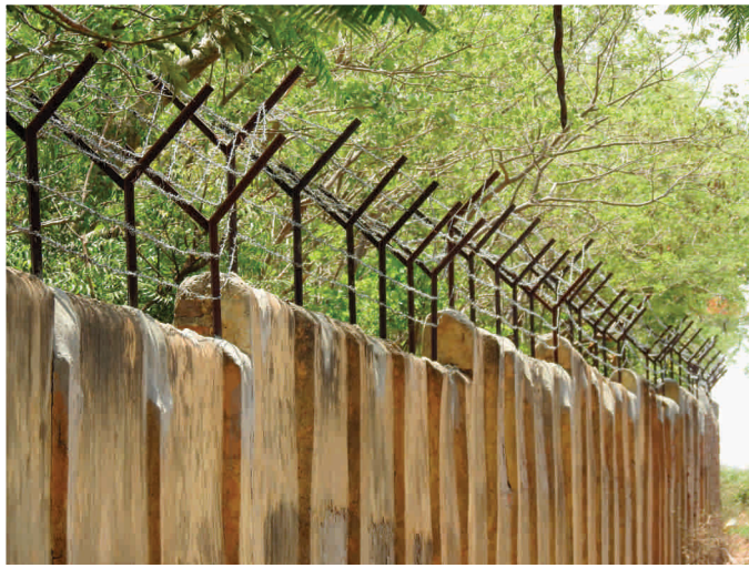
Barbed wire Fencing
