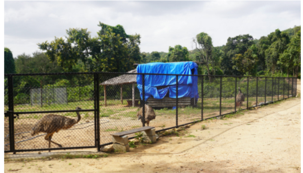
An isolation unit has been established at BBP within the Herbivore Safari to temporarily shift new, sick or injured individuals. This facility enables close observation and effective monitoring while minimizing the risk of disease transmission
