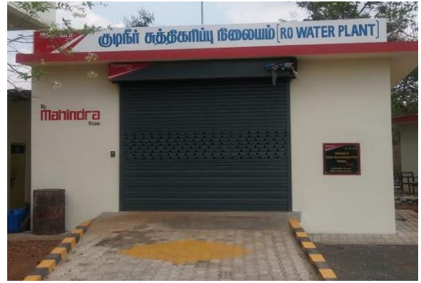
Centralized RO Unit (CSR Sponsored)
