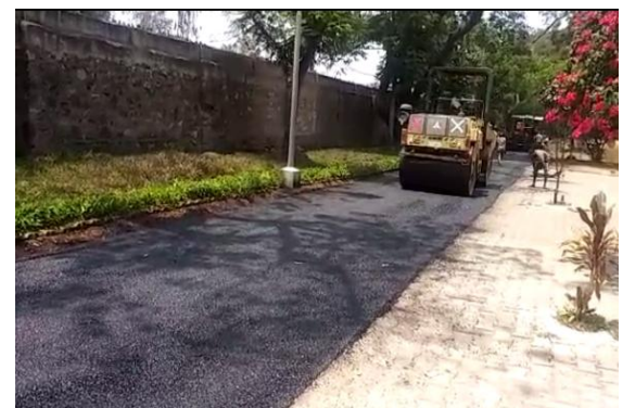
Black topping of Roads
