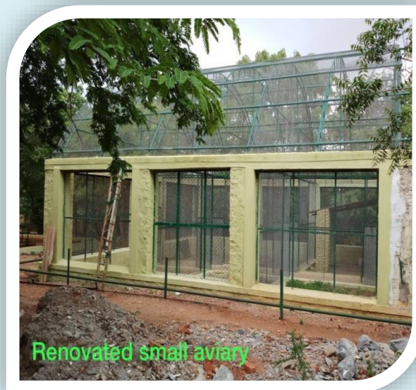
d) Renovated Aviary (2006-17)
