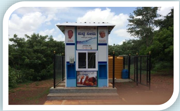
f) RO plant (2016-17)
