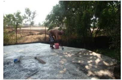
Painting lime to roof of animal house.
