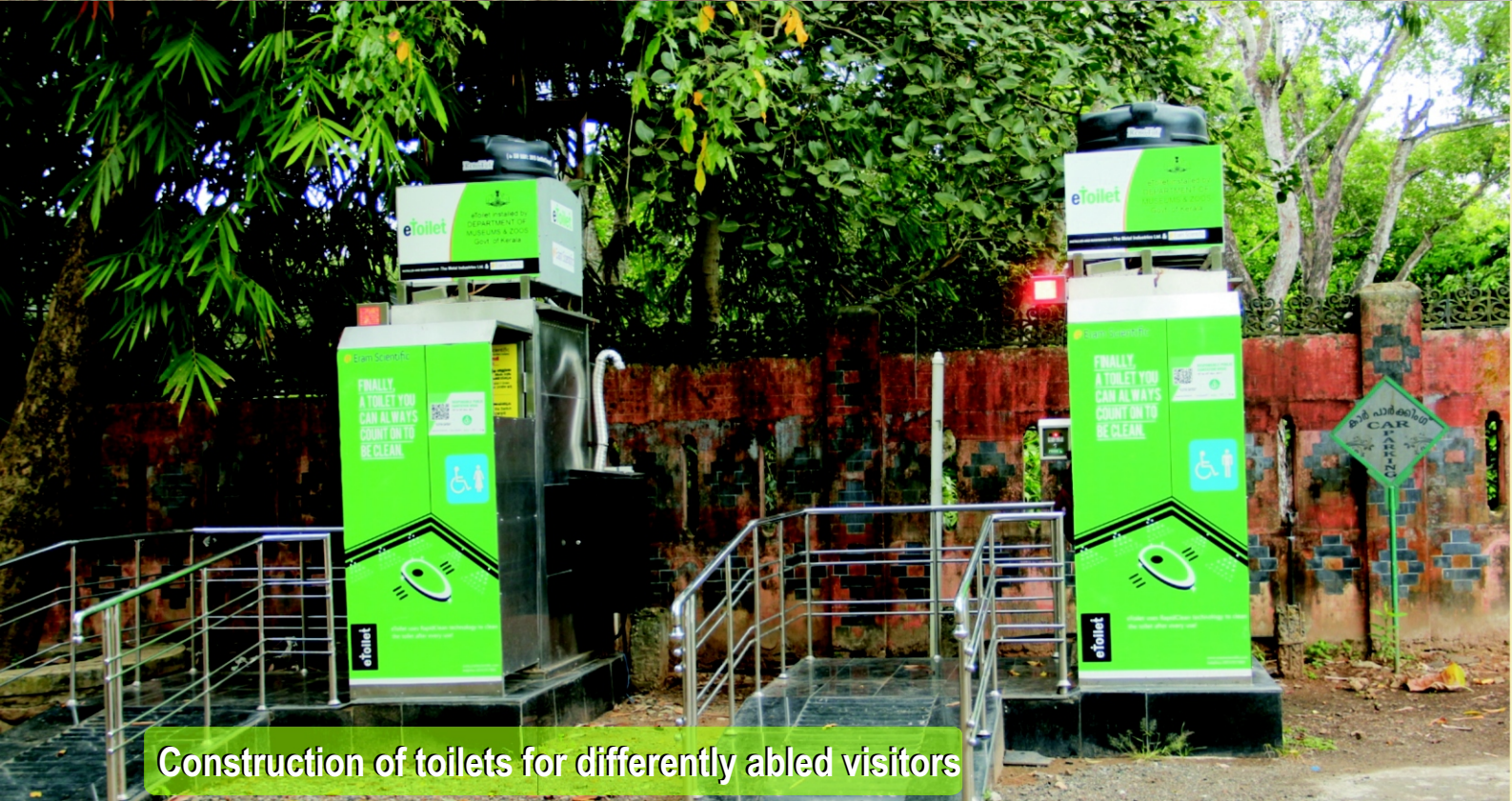
Construction of She Toilets
