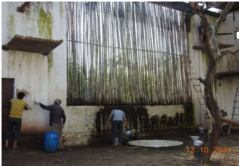
Scrubbing walls to remove fecal matter as well as algal growth
