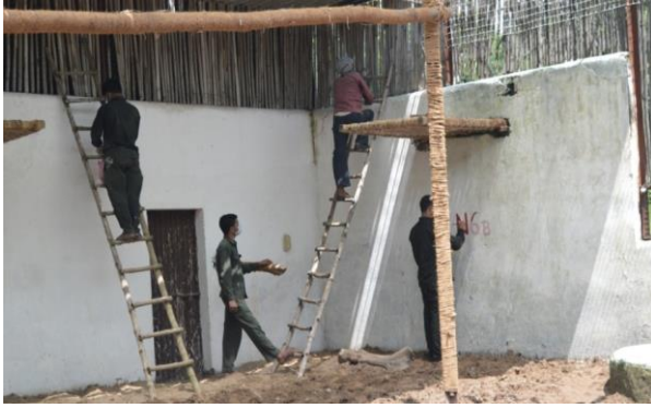
Scrubbing and disinfecting walls with lime
