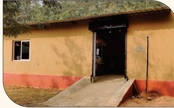
Repairs to Sloth Bear enclosure & Construction of Ice Cream Parlour
