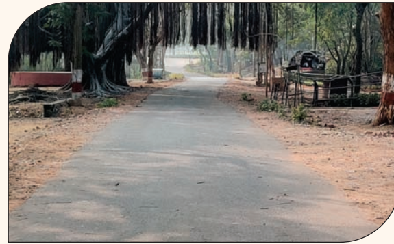
Repairs to BT Road ➔
