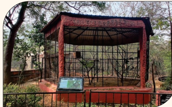
Repairs to Marmoset & Bonnet Macaque Enclosure
