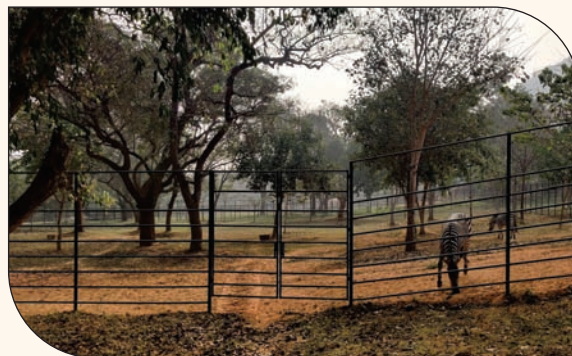
Repair to Zebra Enclosure
