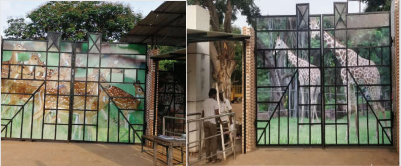
Fabrication of the existing main gate (front) with ACB sheet (heavy duty) IGZP,VSP.
