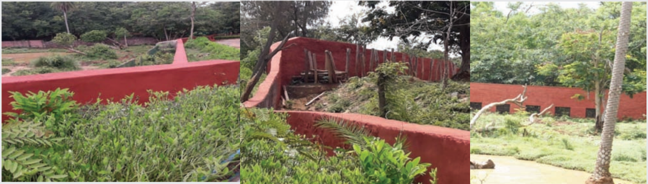
Painting Office building and animal enclosures
