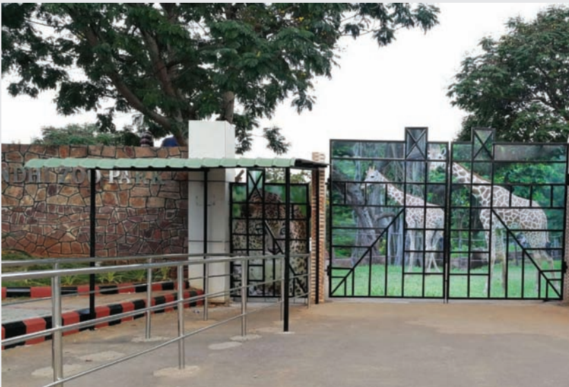
Fabrication of the existing main gate (front) with ACB sheet (heavy duty) IGZP,VSP.
