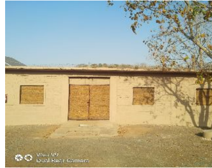
Covered windows and doors with Khus
