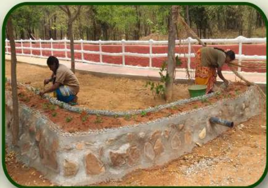
Construction of Saucer Pit at Wild Dog, Hyena and Asiatic Lion enclosures
