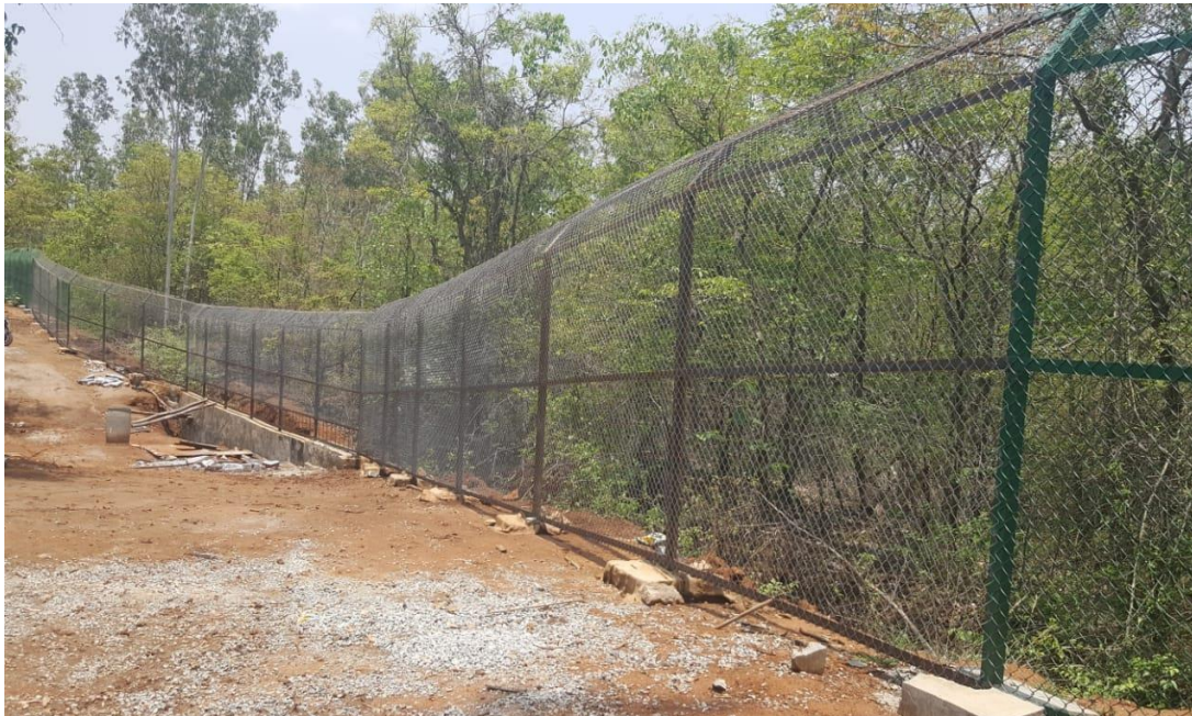
Providing chainlink mesh along the outer boundary of Tiger & Lion Safari, Tyavarekoppa during 2019-20
