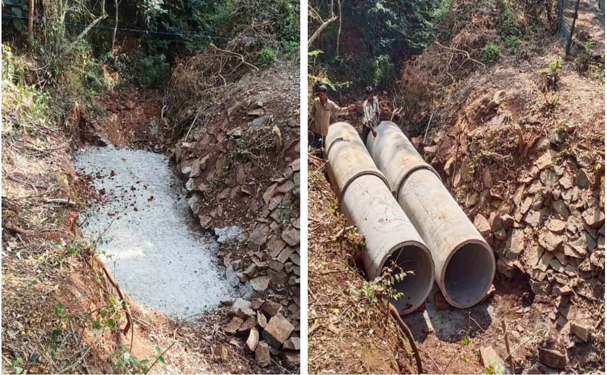
Construction of culvert between Herbivores safari SSM wall & Safari Service road at Tiger and Lion safari Tyavarekoppa, Shivamogga
