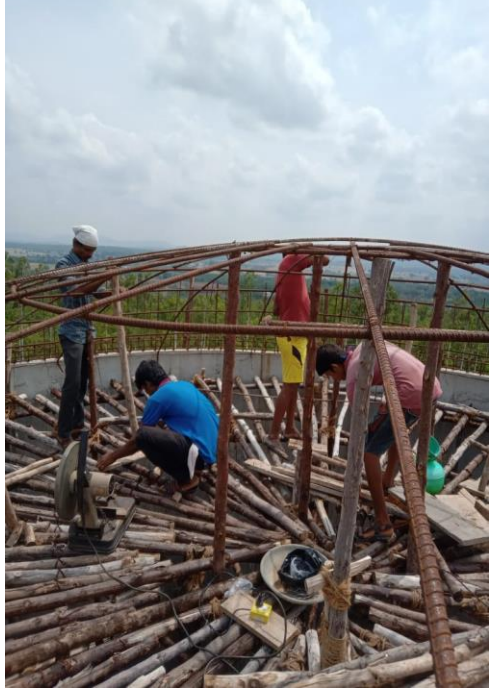
Construction of 2.50 Lakh Litres capacity RCC Intz type Over Head Tank on 15.00mtr staging at Huli Simha Dhama, Tyavarekoppa
