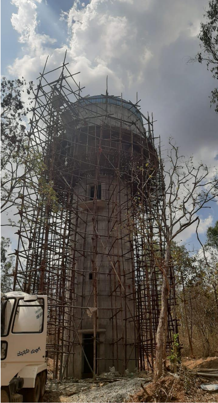
Construction of 2.50 Lakh Litres capacity RCC Intz type Over Head Tank on 15.00mtr staging at Huli Simha Dhama, Tyavarekoppa
