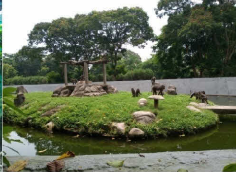
Making of wooden Platform in Mandrill Monkey display area
