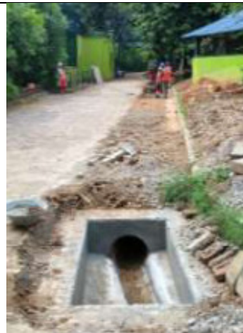
Sewer pipeline laying
