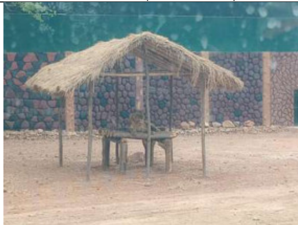
Erection of shade for African lion enclosure
