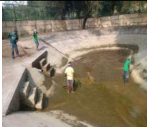
Desilting and cleaning of the pond in the Crocodile enclosure.
