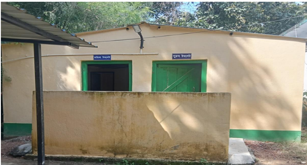
Construction of Visitor Toilet
