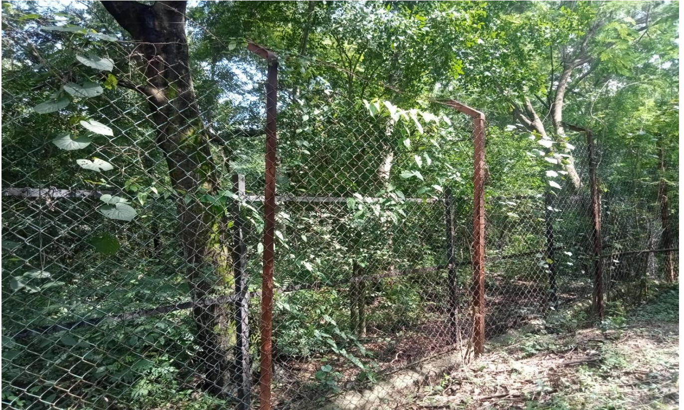
Construction of Sambar Deer Enclosure
