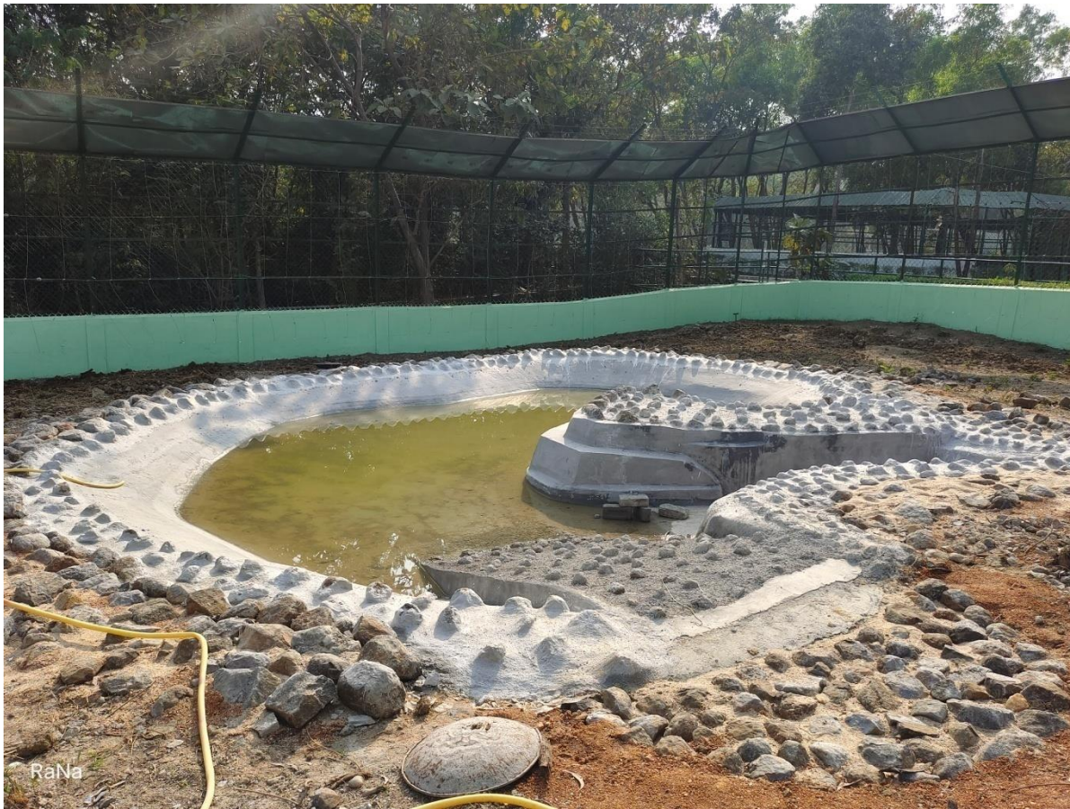
Construction of Leopard Enclosure
