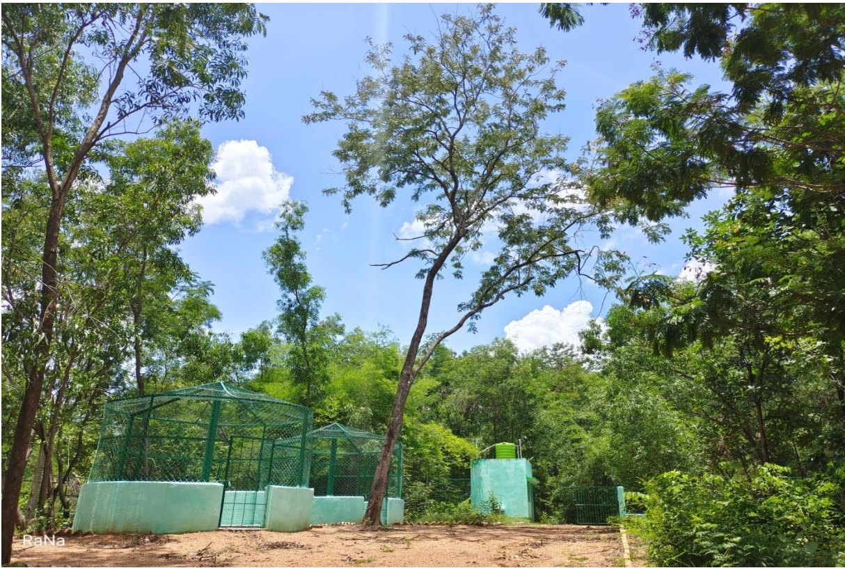
Construction of Rescue Centre
