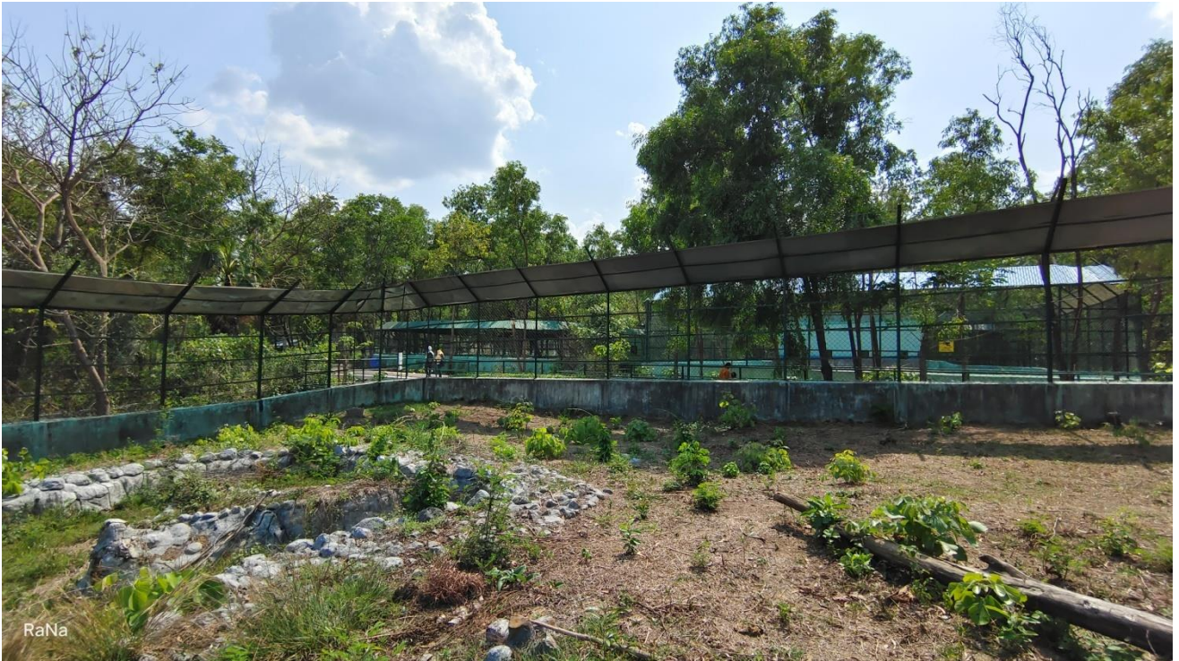
Construction of Leopard Enclosure
