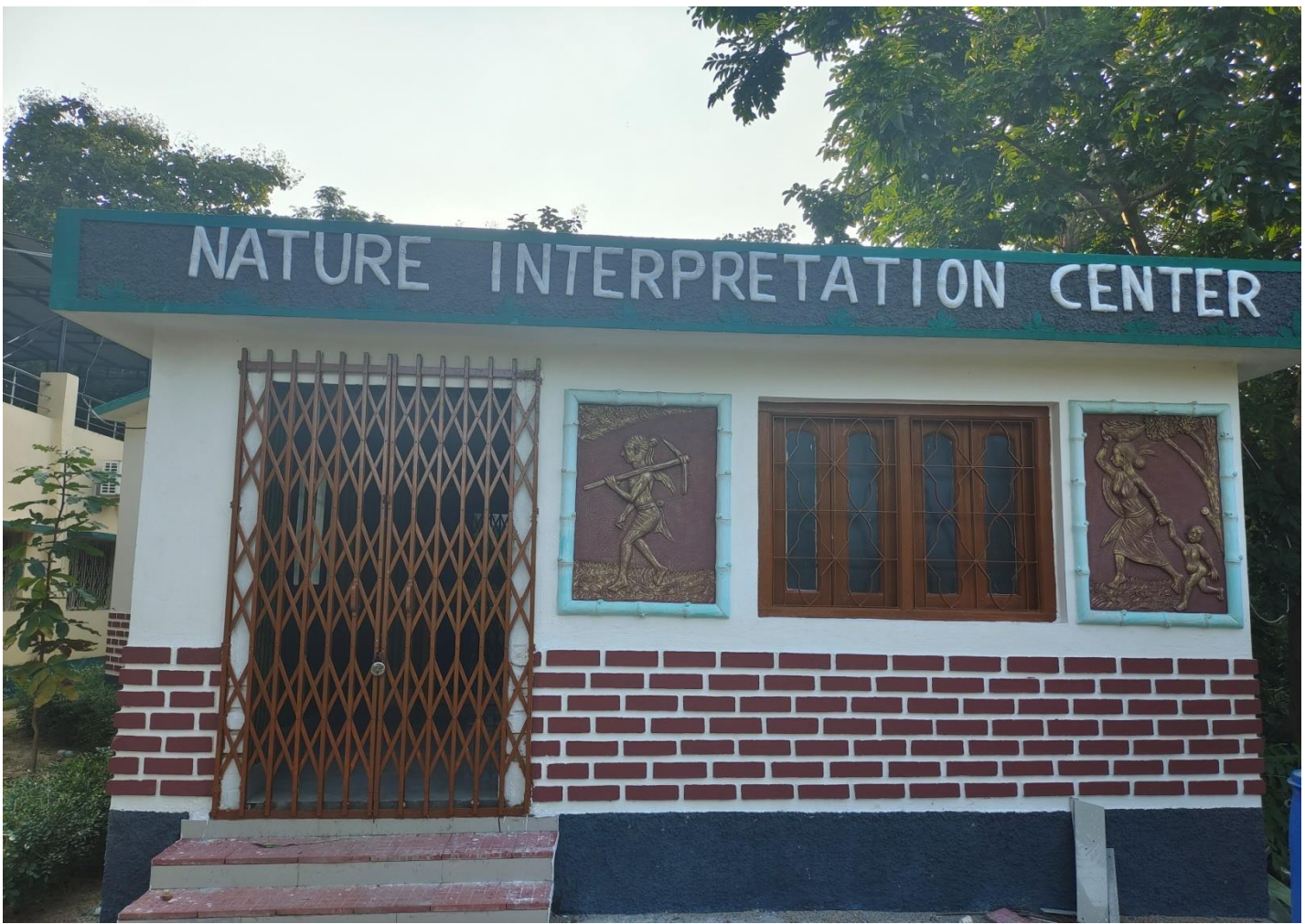
Renovation of NIC Building
