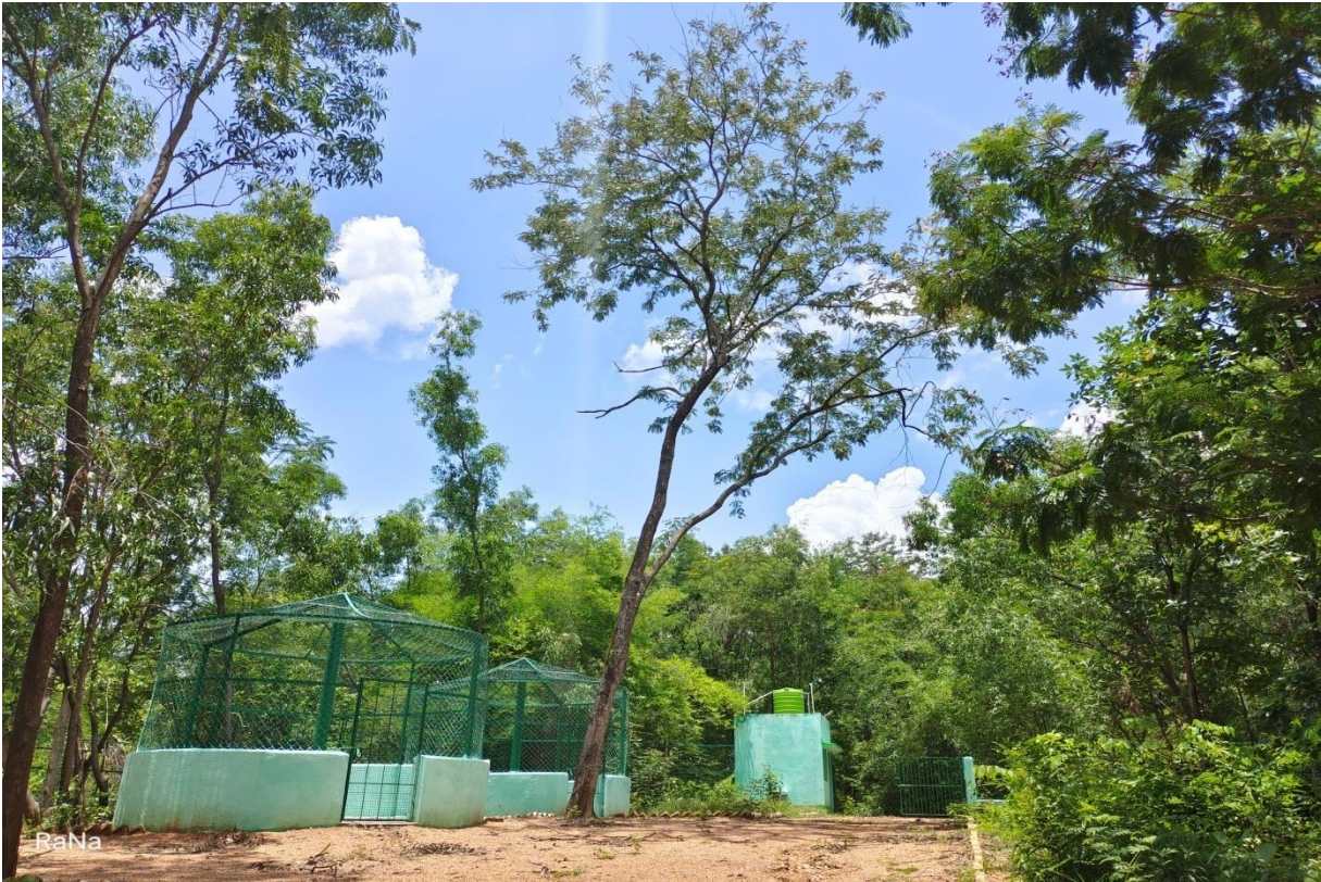
Construction of Rescue Centre
