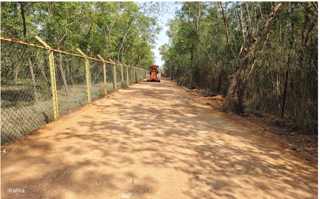
Construction of Service Road
