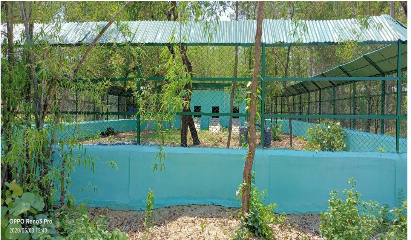
Construction of Hyena Enclosure
