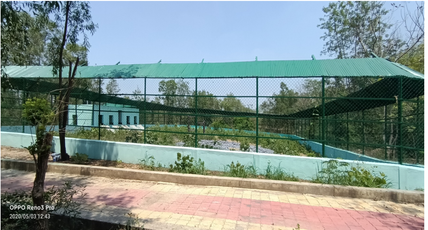
Construction of Leopard Enclosure
