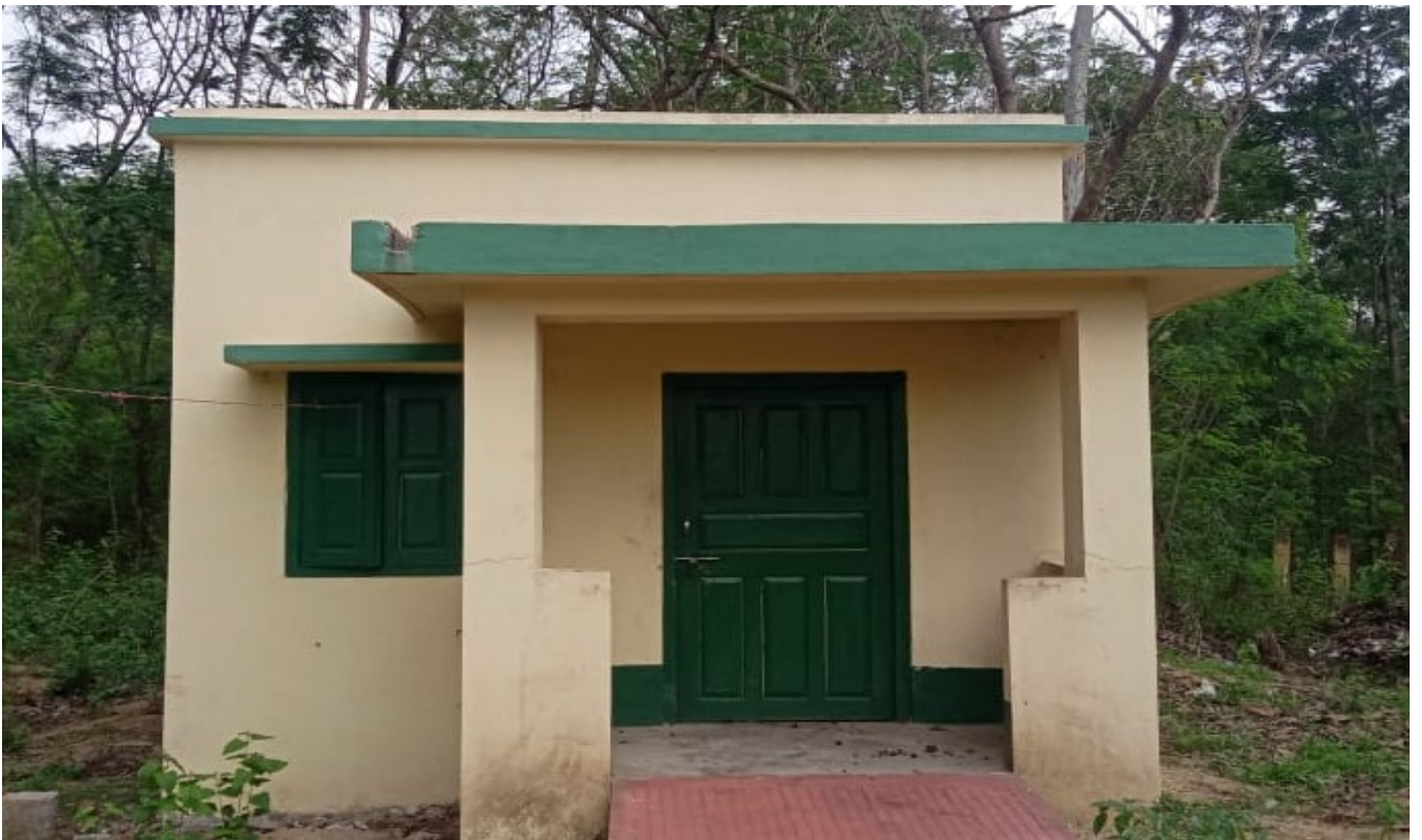
Construction of Post Mortem room
