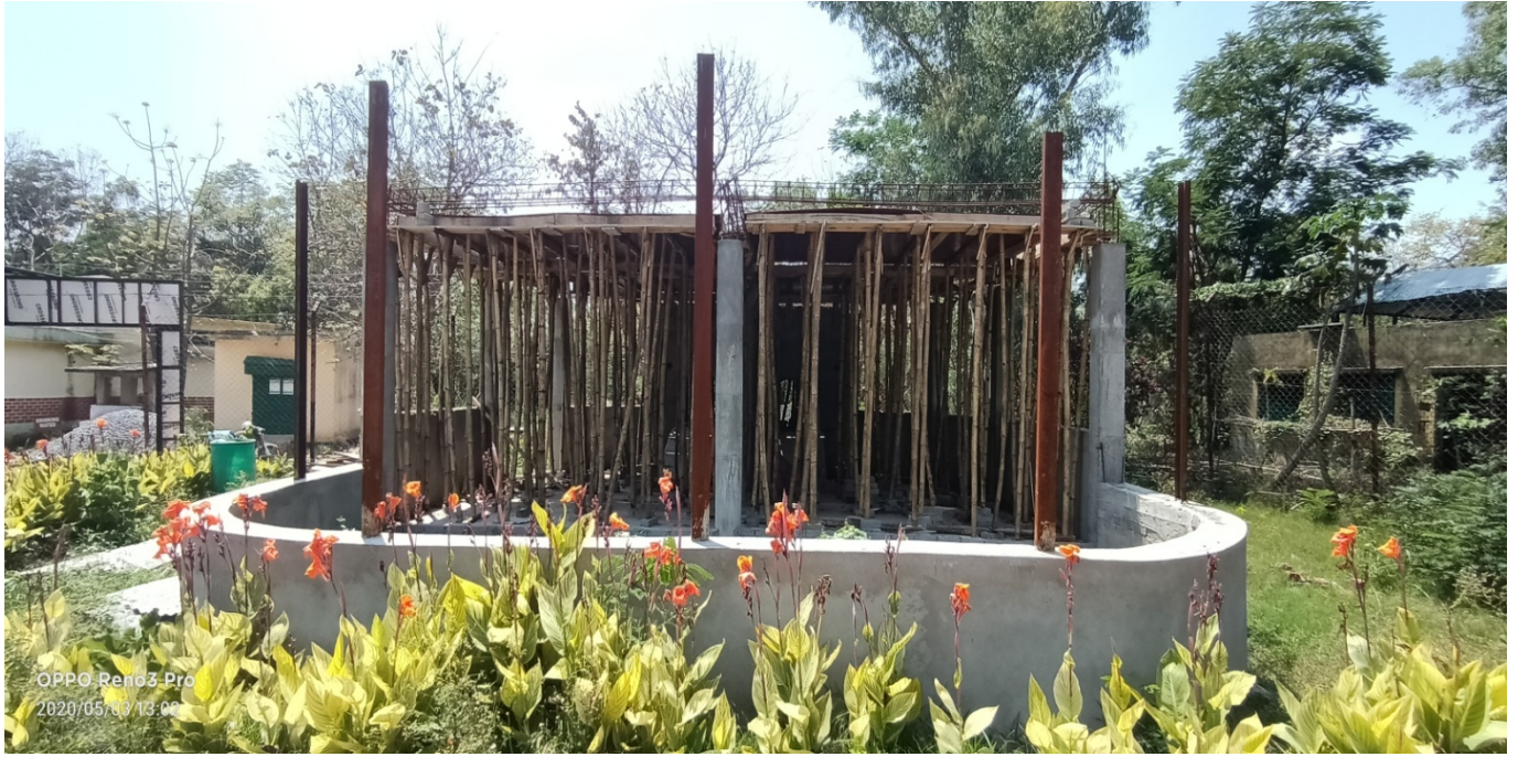
Construction of Porcupine Enclosure
