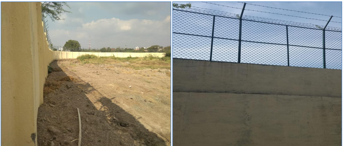
Figure: 2 -construction of RCC wall is completed
