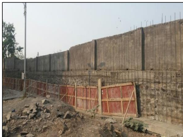
Figure: 2 -construction of RCC wall compound is under process
