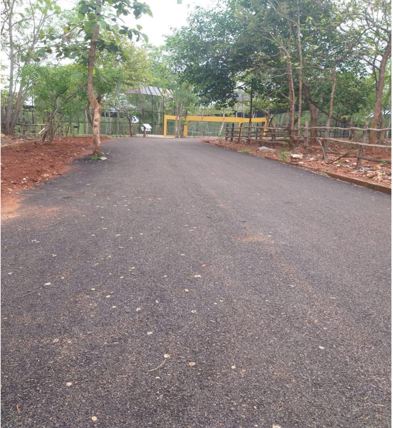
Construction of Road in Zoo path (Chainage 0.0.00 to 807.00= 807.00m)
