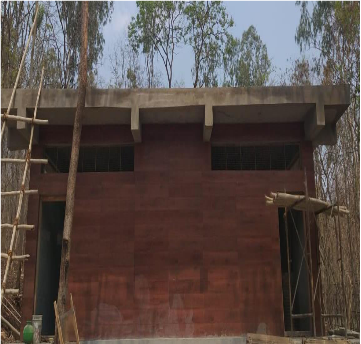
Construction of Toilet Block near Museum
