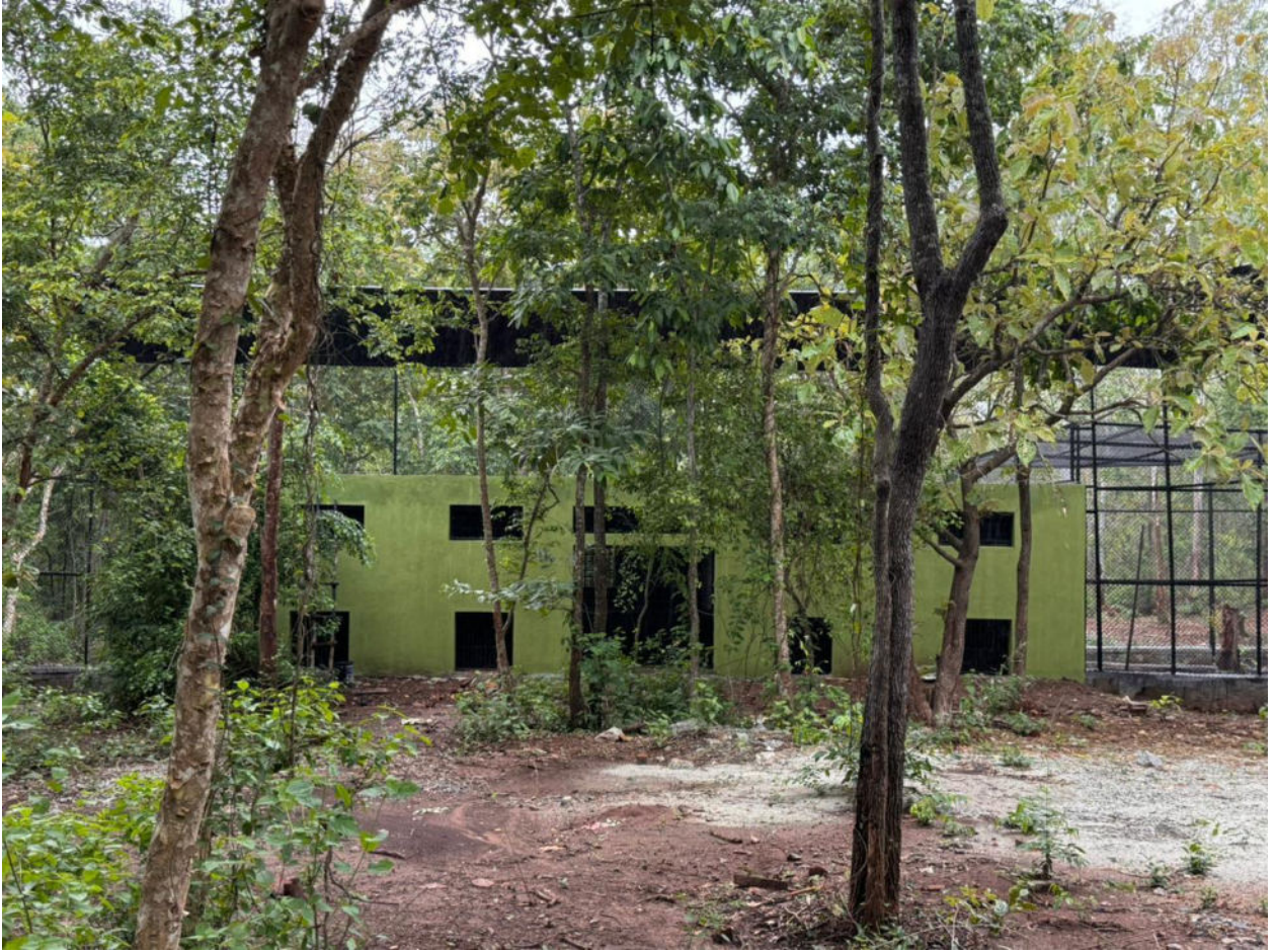
Construction of Lion tail macaque enclosure and holding house
