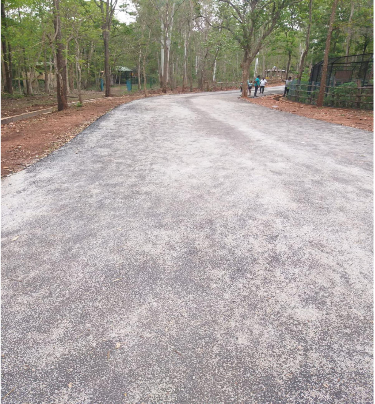
Construction of Road in Zoo path (Chainage 808.00 to 1400.00= 593.00m)
