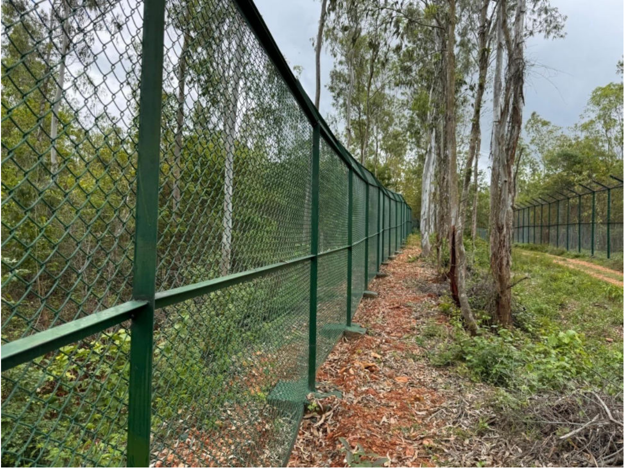
Providing Chainlink Mesh along the outer boundary (Block IV : 1330.00 to 2920.00m)
