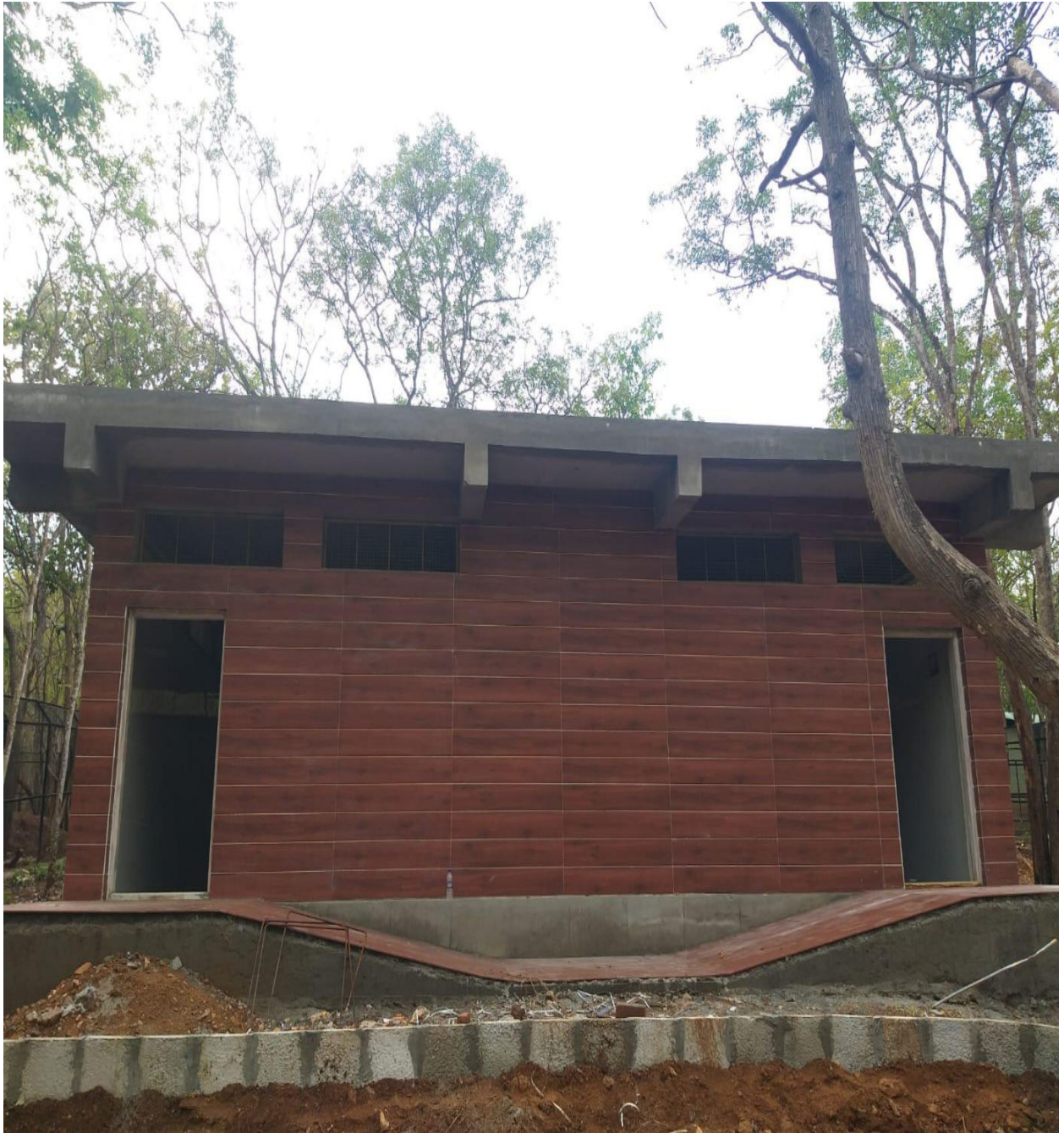
Construction of Toilet Block near Hyena enclosure
