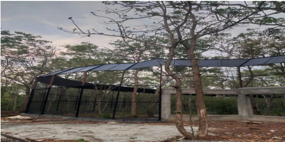
Construction of Common Langur enclosure and holding house
