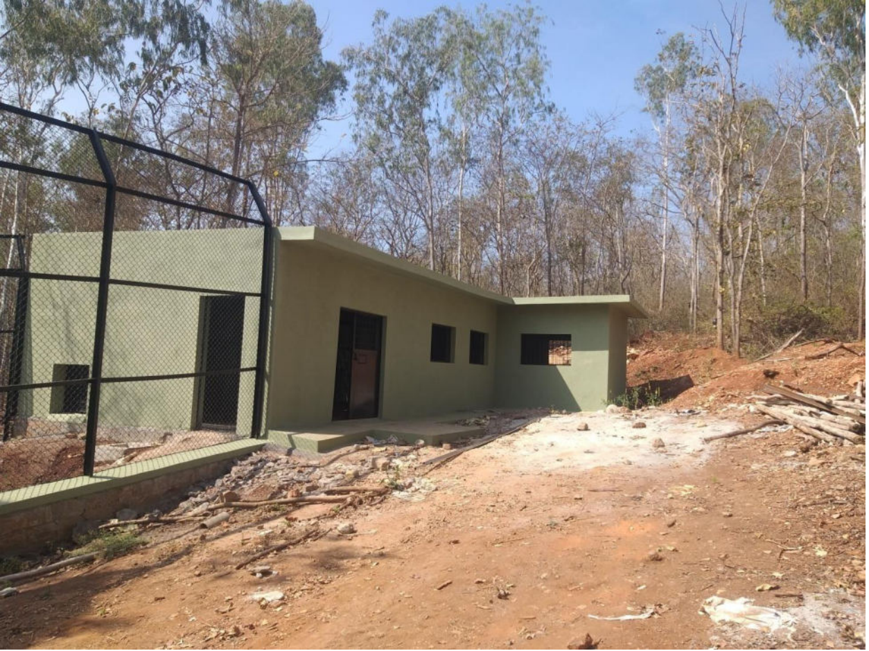
Construction of jackal enclosure and holding house
