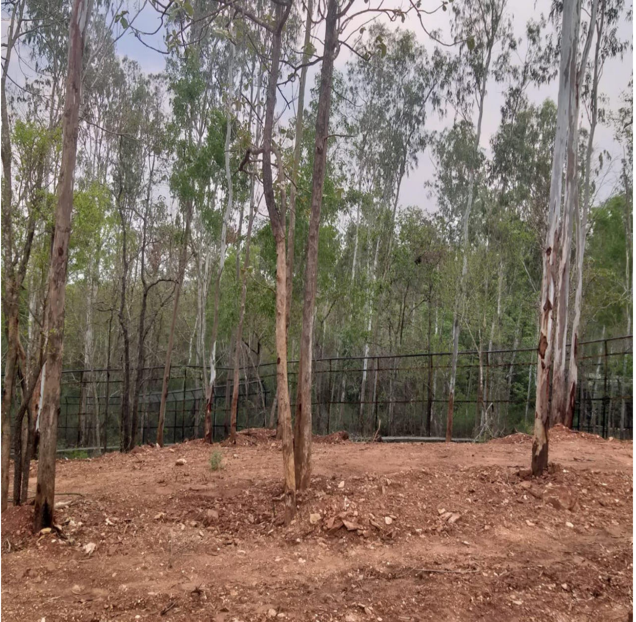
Construction of Zebra enclosure and holding house
