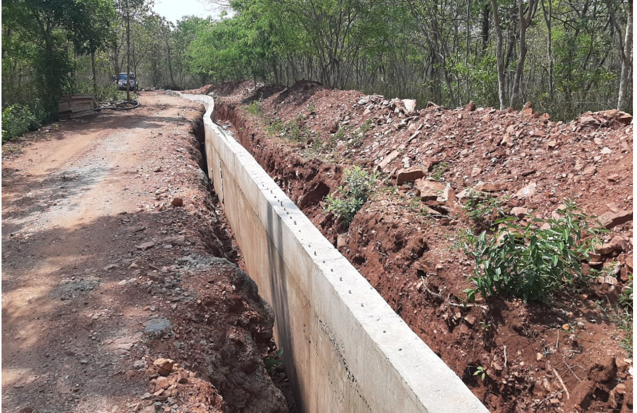
Construction of INDIAN GAUR Enclosure, holding house is in progress
