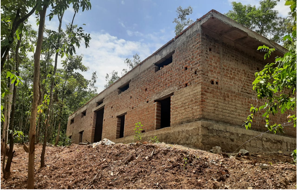
Construction of TIGER enclosure and holding house is in progress
