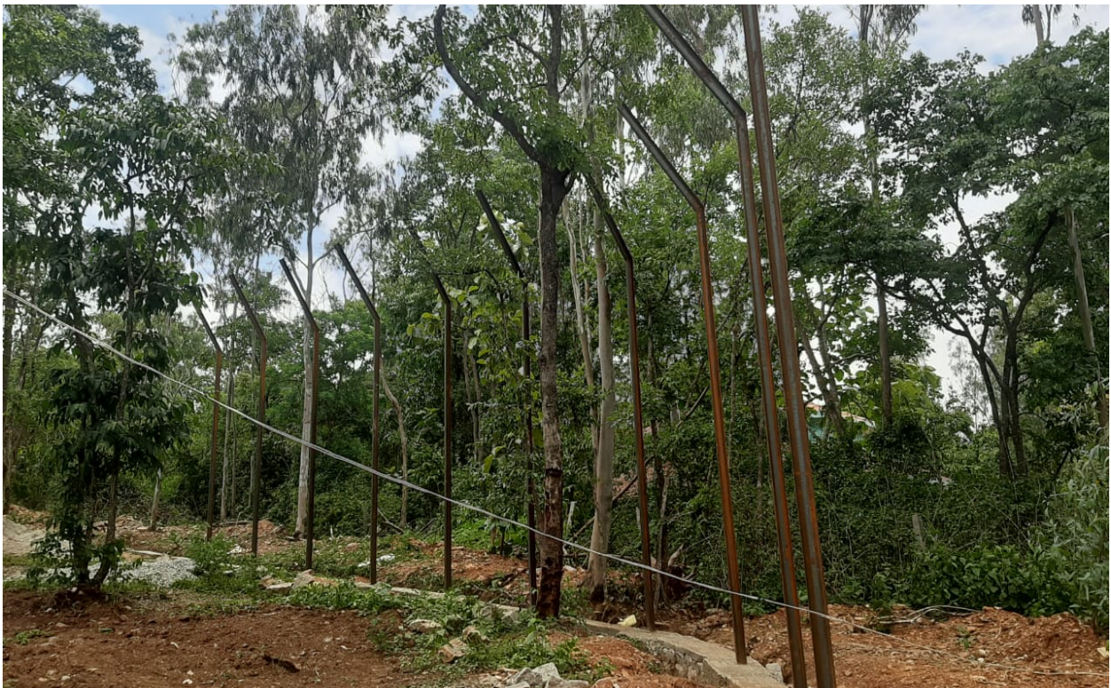
Construction of LEOPARD enclosure and holding house is in progress
