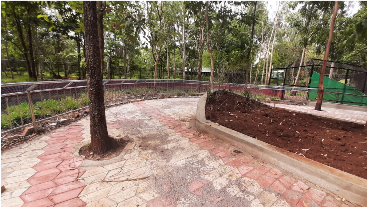
Construction of Ostrich enclosure
