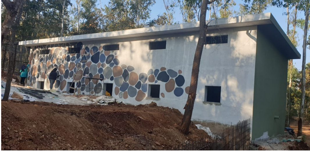
Construction of enclosure for Hyena
