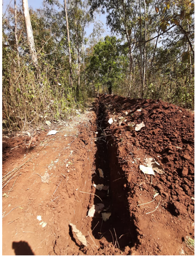
Laying of feeder main from OHT to zoo enclosures is in progress
