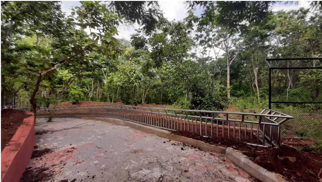
Construction of Spotted deer enclosure
