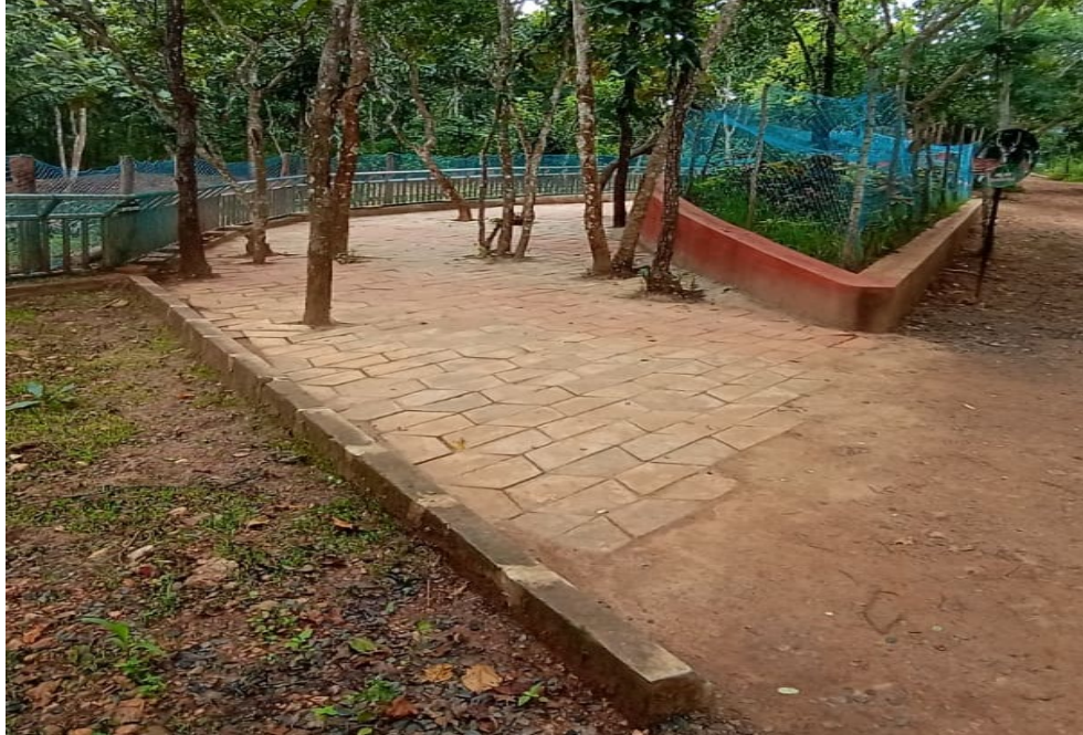
Construction of Nilgai enclosure
