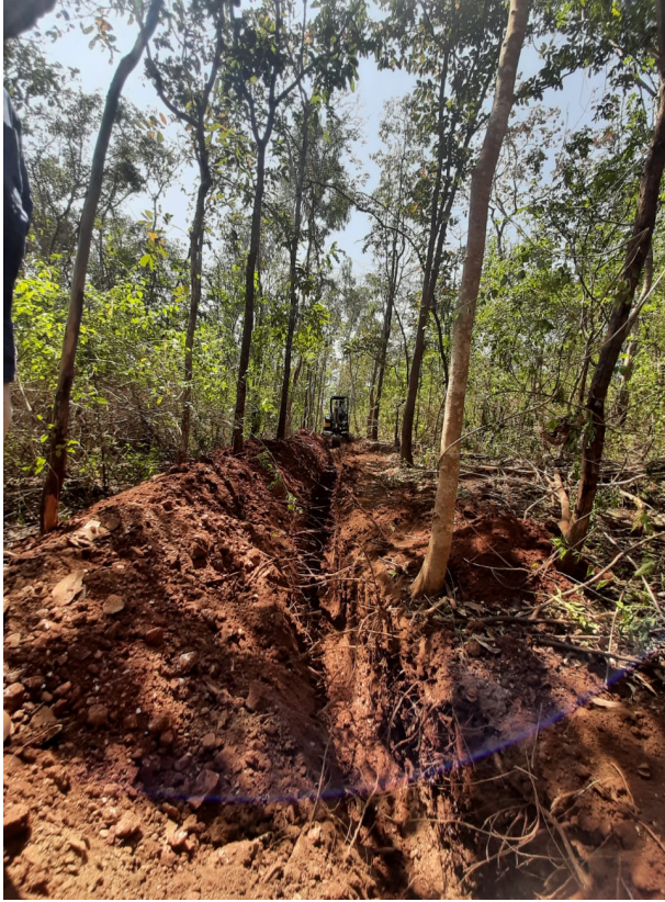
Laying of feeder main from OHT to zoo enclosures is in progress
