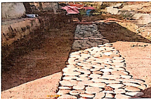
17. Laying of paver tile at main gate.
