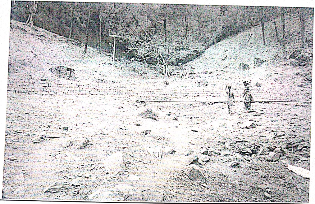
4. Construction of Check walls.
