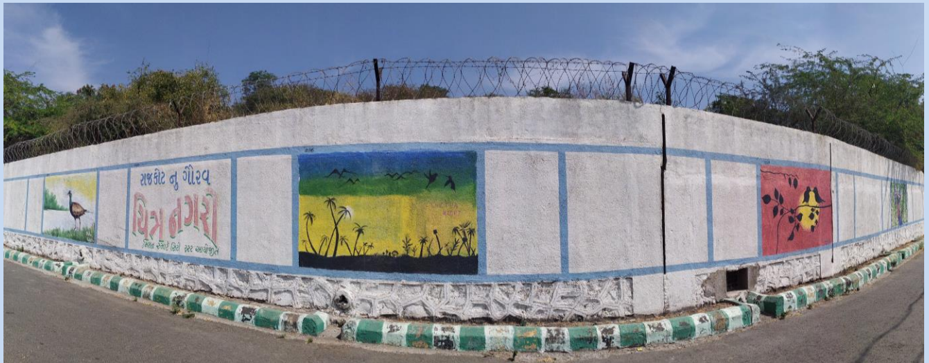
Concertina Coil on Rajkot Zoological Park Perimeter Wall
