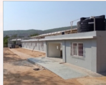
Sufficient number of windows for ventilation in Retiring room
