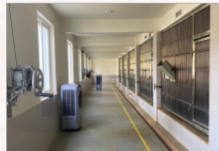
Interior of Retiring Room- SS Cells, CCTV Cameras for monitoring, Use of Kota in Keeper's Gallery, Gear-Box based drop gate lifting mechanism and Post Box feeding window
